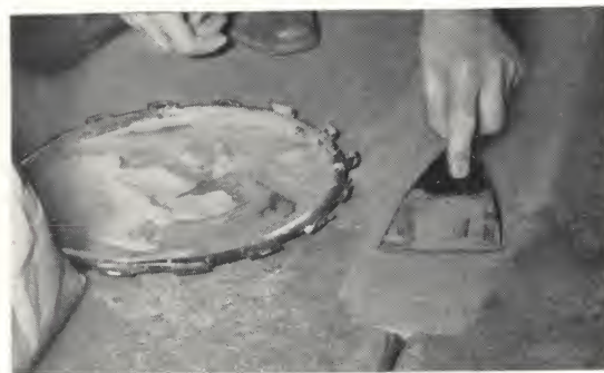
Although resilient flooring adhesives will fill minor cracks and crevices in concrete subfloors, it is best that all conspicuous holes, cracks, and crevices be filled with a reliable cement crack filler before installation is started. It is important that all concrete subfloors be allowed adequate drying time before installing flooring.
