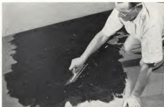
Latex-type underlayments may be troweled to a thin "featheredge" in leveling worn or damaged areas of concrete subfloors. This often eliminates the need for grinding or a complete new concrete topping.
