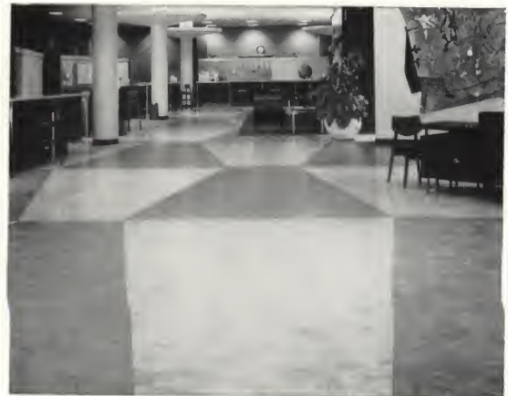
More elaborate custom styling as in the floor above costs more than that on the left due to increased cutting and fitting. Curves and irregular shapes would cost even more.
