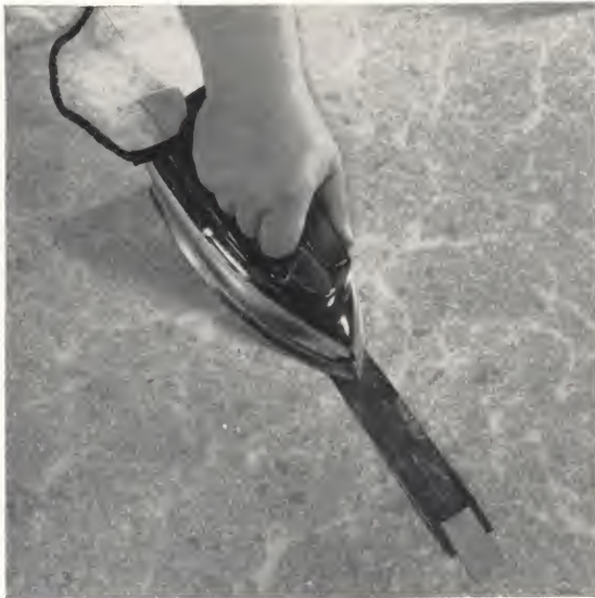
An electric iron and aluminum foil in experienced hands can weld seams in vinyl sheet flooring and, by eliminating dirt traps, create a "cleaner," more cleanable floor.
