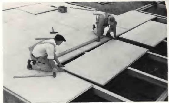
Among the advantages of 2-4-1 T & G Plywood are: fewer individual pieces to handle, register holes can be cut without framing, fewer joints for air drafts, less labor and material costs, uncluttered basement ceilings, and no underlayment needed beneath resilient flooring.
