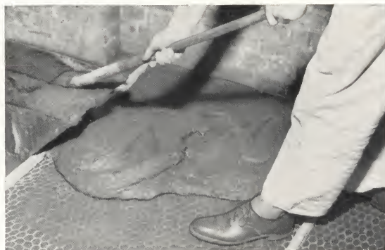
Over wood subfloors, galvanized chicken wire or expanded metal lath should be nailed to the floor to reinforce asphaltic-type underlayments. The wire mesh allows the wood floor to expand and contract without damaging the floor fill.
