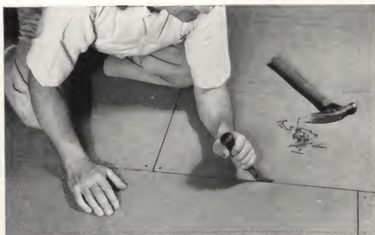
Hardboard or plywood (joint spacing of \frac{1}{32} ") should be fastened to the subfloor with coated or ring-grooved nails or approved staplers. Fasteners must not be over 4" o.c. in all directions and at edges and driven flush or \frac{1}{32} " below the underlayment surface.
