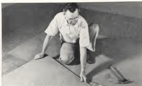
An underlayment, consisting of four-by-four sheets of approved hardboard or plywood, is advised for rough wood subfloor areas which cannot readily be corrected by sanding. When laid over a tongue-and-groove floor, these underlayments provide a sound and economical base for all types of resilient flooring.
