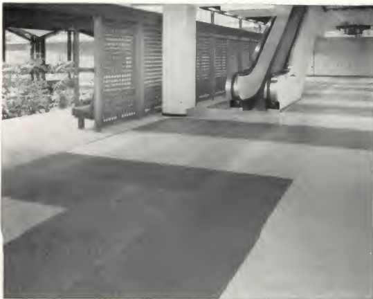
Custom floor designs can be achieved without greatly increasing the cost. Right angles, straight lines, and minimal waste made this striking custom floor cost very little extra.
