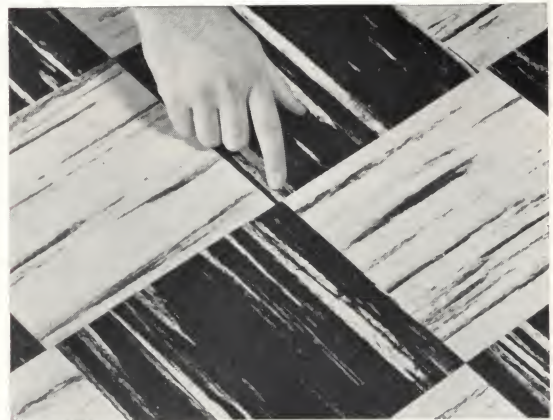
All joints or seam lines should be symmetrical. Uneven lines, such as illustrated above, are more likely to occur in tile installations. Armstrong resilient tiles are die-cut to a perfect square to avoid this condition providing the flooring mechanic squares the room and lays the tiles carefully.
