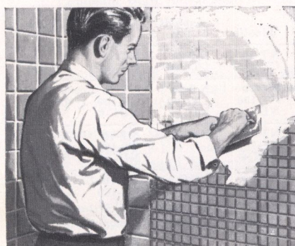
1. Grout-adhesive is applied to the foundation board with a plasterer's trowel, filling grooves and leaving a thin film of grout-adhesive on the raised surfaces.
