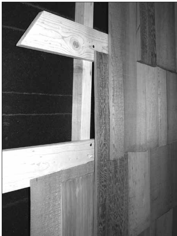
Figure 8. Rain screen technique.
