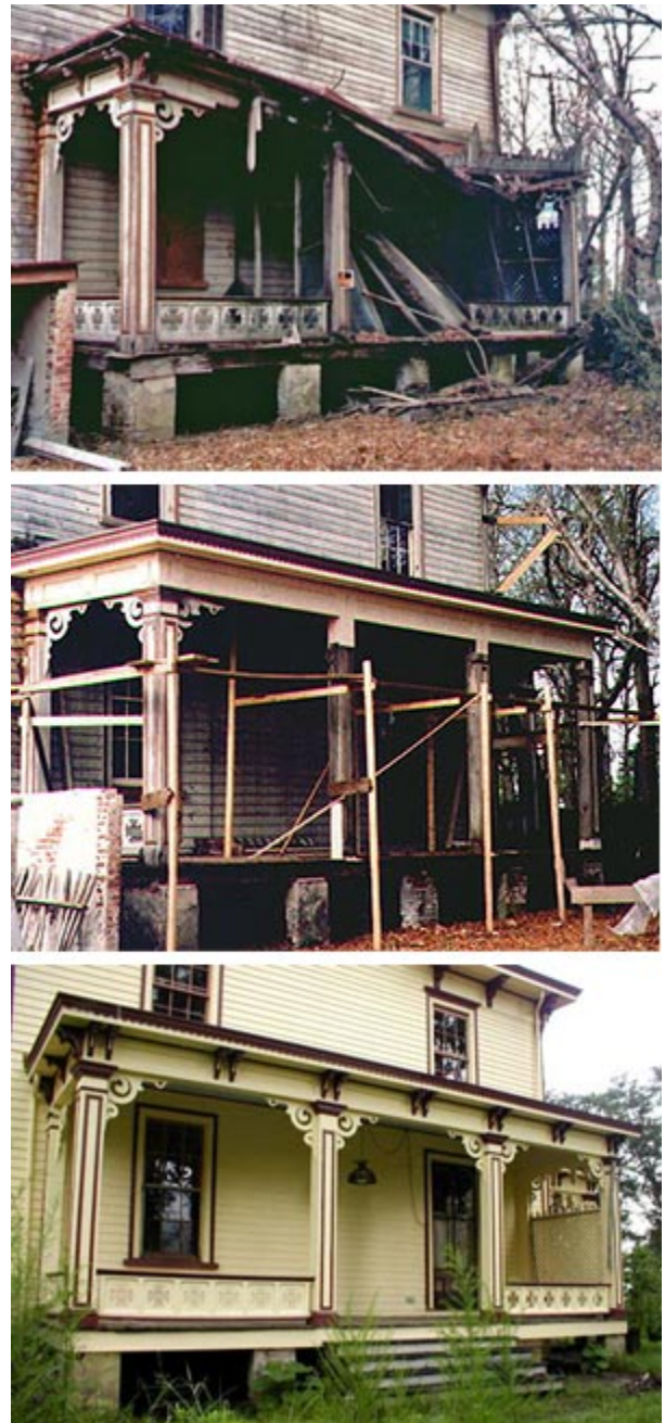
Figure 5. Even historic porches that appear to be in total disrepair may be repairable. While the roof needed replacement, much of this porch was repaired, including such features as the decorative columns, ornamental brackets, and balustrade. Photos: John Leeke.
