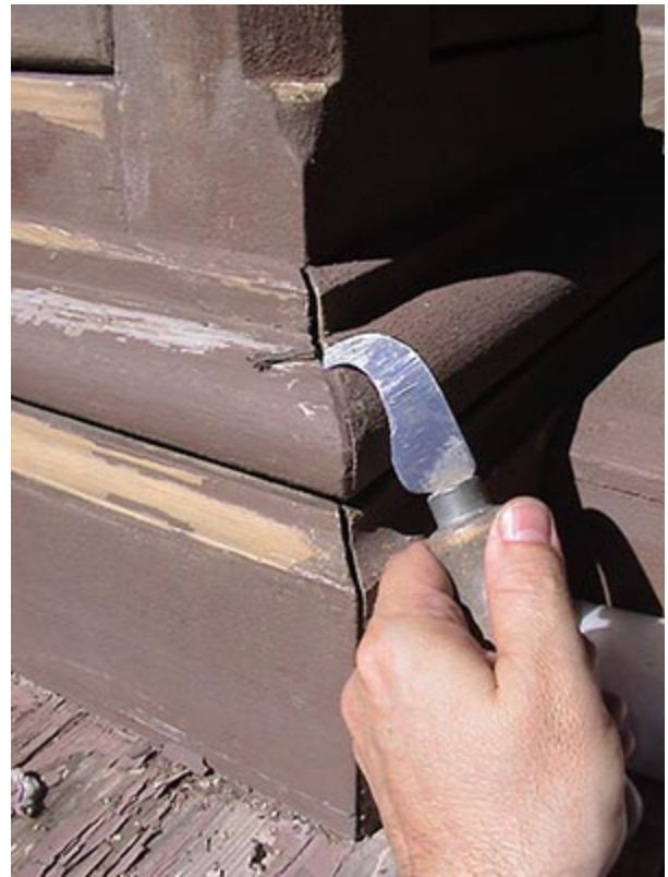
Figure 7. Common problems with porches that can contribute to serious wood decay include cracks in woodwork and joints that have opened up. Both provide an easy path for water seepage. Trapped moisture can foster peeling paint, wood decay and insect infestation. Open joints and cracks should be checked for evidence of more serious decay and marked for caulking or repair. Photo: John Leeke.
