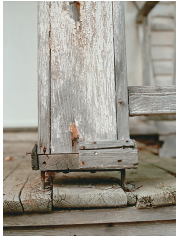
Figure 6. A traditional way to extend the life of porch posts was to place posts on metal feet, thereby providing a separation between the wood post and wood deck. This helped to prevent the wood post from rotting at the base. Early post feet were simple iron bars bent unto a stirrup shape. By the late nineteenth century manufactured cast-iron feet were common, consisting of a pair of disks separated by a short pipe. Post feet are still available today. Courtesy of Old-House Journal/Brian McNeil.
