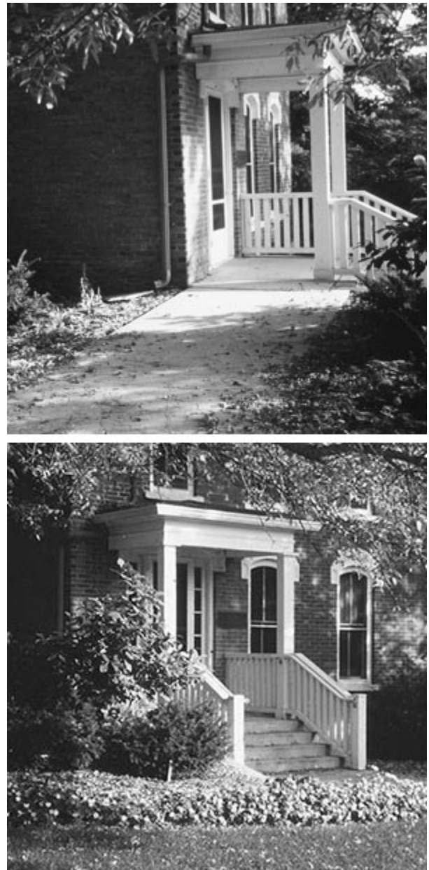
Figure 18. When a porch is used as a wheelchair accessible entrance, it may be possible to retain the historic stairs by adding a ramp parallel to the building. Through plantings and some re-grading, the new ramp built parallel to the building (left) allows retention of the historic stairs and does not impact the historic character of the entrance (right). Photo: Iowa State University Extension.
