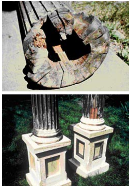
Figure 10. This nineteenth century porch column is made of wood staves, similar to the way a wood barrel is put together. After replacing the torus and making dutchman repairs to the apophyge along the base, the column and pedestal are ready to be reinstalled on the porch. Photos: NPS files.
