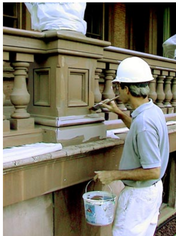
Figure 8. Decay can start when wood is left exposed to the weather or where joints open up. An inexpensive way to extend the life of the existing porch paint without jeopardizing the historic material is spot paint and caulk where needed every year or two. This cost-effective procedure is particularly effective in maintaining wood porches where the exposure to weathering is high. Photo: John Leeke.
