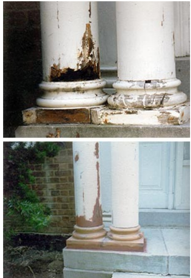
Figure 11. The lower shaft of the porch columns had decayed as water wicked up through the end grain (top). The column shafts were repaired in place by cutting out the deteriorated wood and making repairs using epoxy consolidants and fillers. (bottom). The column bases were replaced. Photos: Paul Marlowe, Marlowe Restorations.
