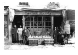
Virginia had an operable awning retracted against the building facade. Hinged extension arms were raised and lowered allowing for an awning configuration easily changed in response to weather conditions. This photo shows how the fabric gathered and was exposed to the elements when retracted - part of the reason roller awnings later became prevalent. Photo:
