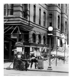
frames. Here, a pipe frame without its canvas cover extends around the corner of a building in Washington, D.C. Photo:
