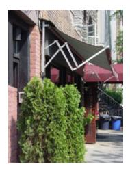
Lateral-arm awnings were preferred on long elevations, especially those with sheet glass (where vertical arms could not be fastened to the building façade). When lateral arm awnings were installed across a broad storefront or porch, manufacturers recommended spacing the arms at approximately eight
