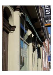
awning had a large projection, extending far from the building wall, the lower hinges were mounted on vertical slide rods affixed to the facade. When the awning is lowered, the bottom hinges of the arms travels up the slide rod to increase headroom beneath the fully extended awning. Photo: NPS files.
