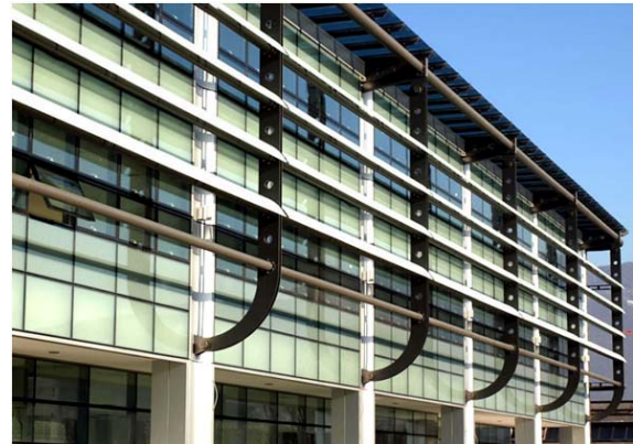
Figure 10. Brise soleil - shading devices integrated with the building facade
