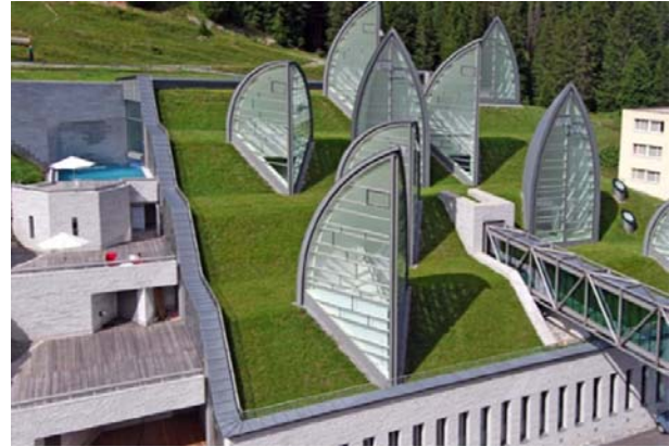
Figure 10. Shading by trees and vegetation (green roof)
