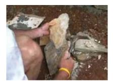
Stones can be reshapped using a chipping hammer.
