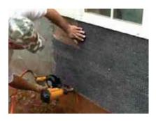
Attach metal lath once the moisture barrier is in place.
