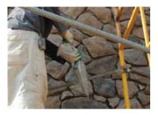
Add mortar to the joints between the stones using a grout bag. Squeeze the mortar into the joints using a twisting motion.
