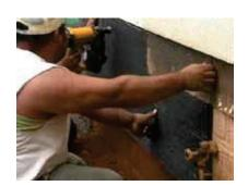
Install a moisture barrier prior to installing stone veneer.
