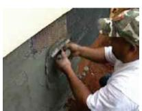
Apply a scratch coat over the metal lath. The mortar should be applied approximately 1/2 inch thick, ensuring the lath is completely covered and in place at least 12 hours before setting stone.
