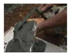
Place a bed of mortar on the back of the stone. Use the trowel to create a space in the center of the mortar to help with adhesion.
