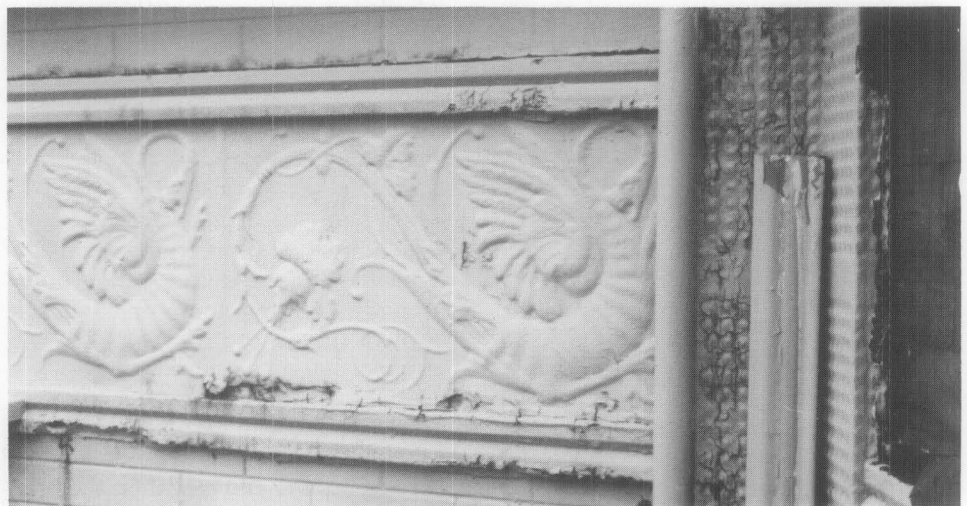
3. Stamped metal siding simulating brickwork covered most of the exterior of the house. Pebbled corner pieces and several ornamental bands added decorative details. Deteriorated drainspout and original plank wall sheathing are at right. Photo: Richard Hiler.
