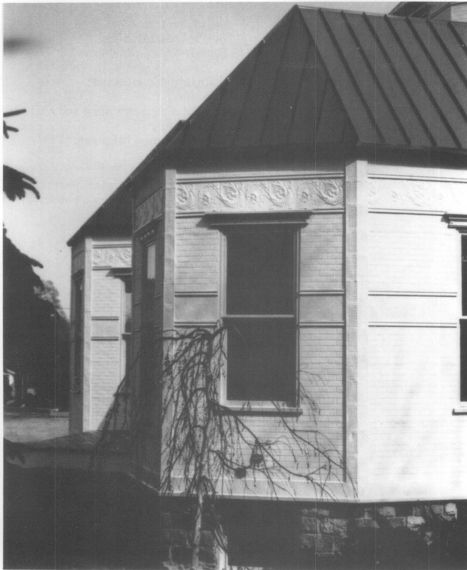
11. Finished appearance of several elevations. Siding has been face nailed to underlying materials and second coat of paint has been applied. Each piece of siding laps over the piece below it, and all overlap the corner pieces. Photo: Richard Neumann.
