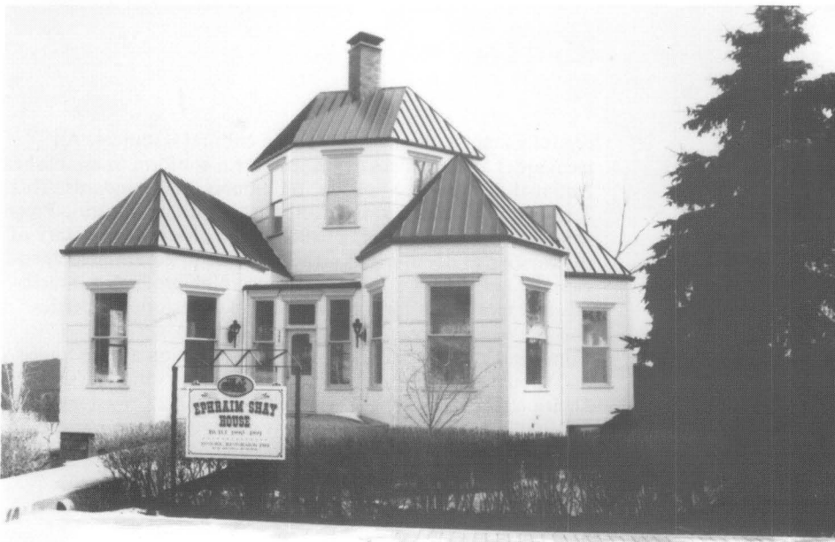
12. The replication of the stamped metal siding has restored the Hexagon to its historic appearance. A new metal panel roof system that duplicates the appearance of the original standing seam roof also contributes to the restoration. Photo: Richard Neumann.
