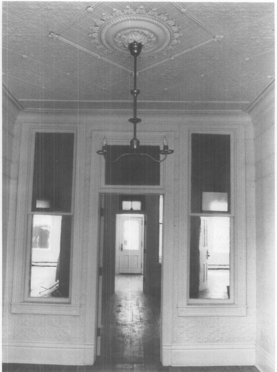
2. The walls and ceilings of each interior room are sheathed with stamped metal siding in a variety of decorative patterns. Photo: Brian Conway.
