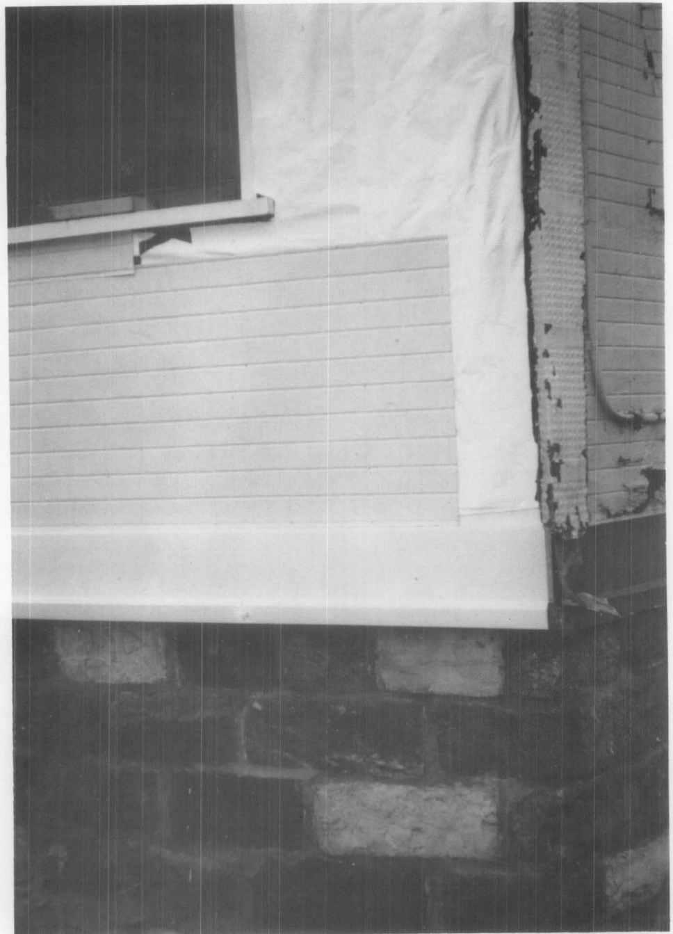
10. Installation of siding began at the base of each story of the building. Corner pieces were installed first, followed by the base flashing, and the stamped brick siding. Care was taken to match the patterns from one elevation to the next around the building. Photo: Mary Cay Bartush Jones.
