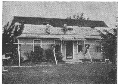
Figure 34. Reroofing over the old shingles saves labor and expense.
