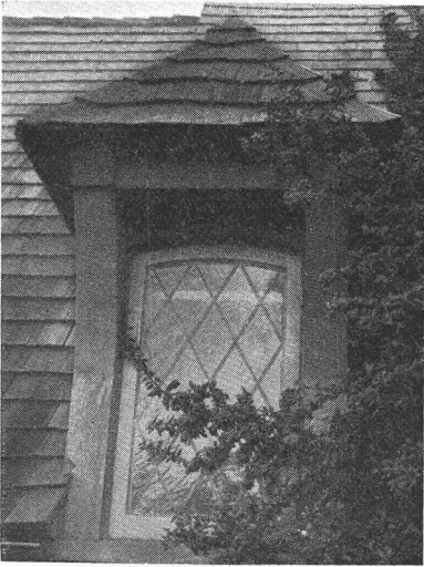
Figure 23. Neat "set in" hip shingle.
