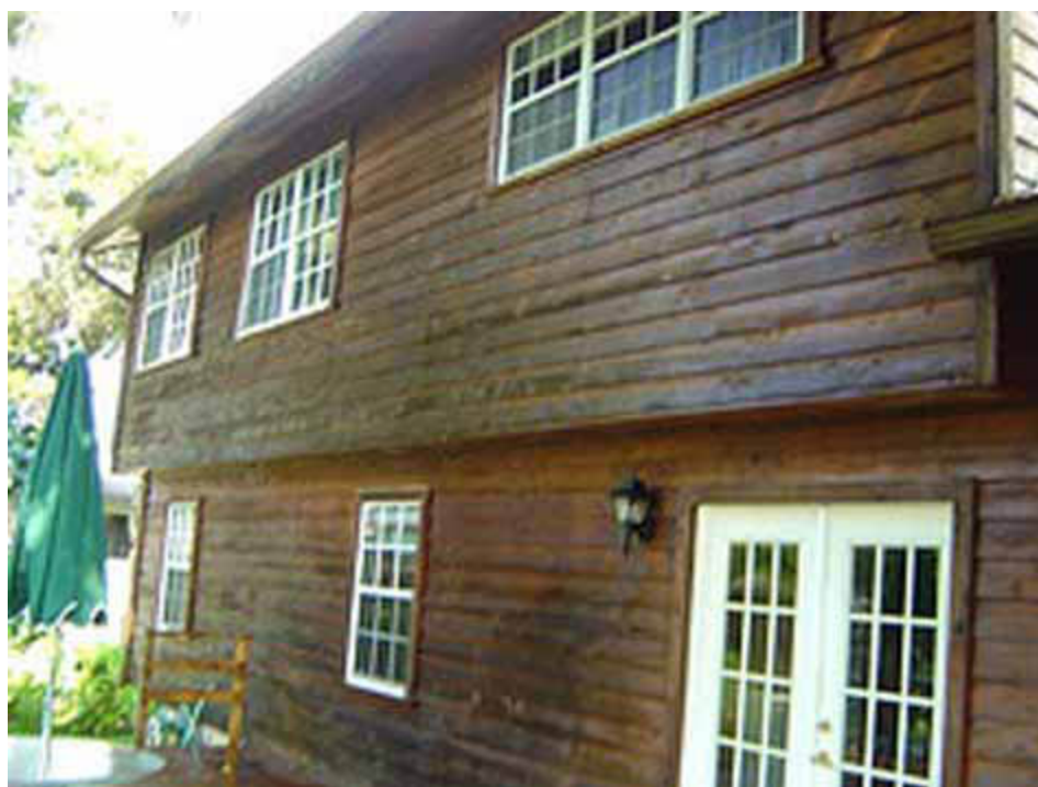
The cedar siding on this house has become stained. Photo from Flickr: https://www.flickr.com/photos/jahluka/
