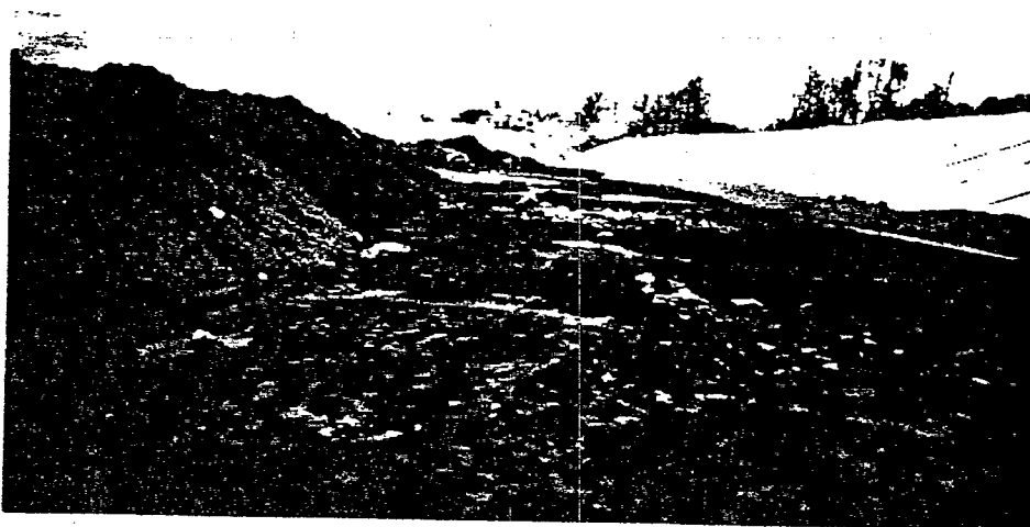
(a) Photograph of the Landfill. A Large Majority of the Waste Consisted of Slurred Fines from an Industrial Process.
