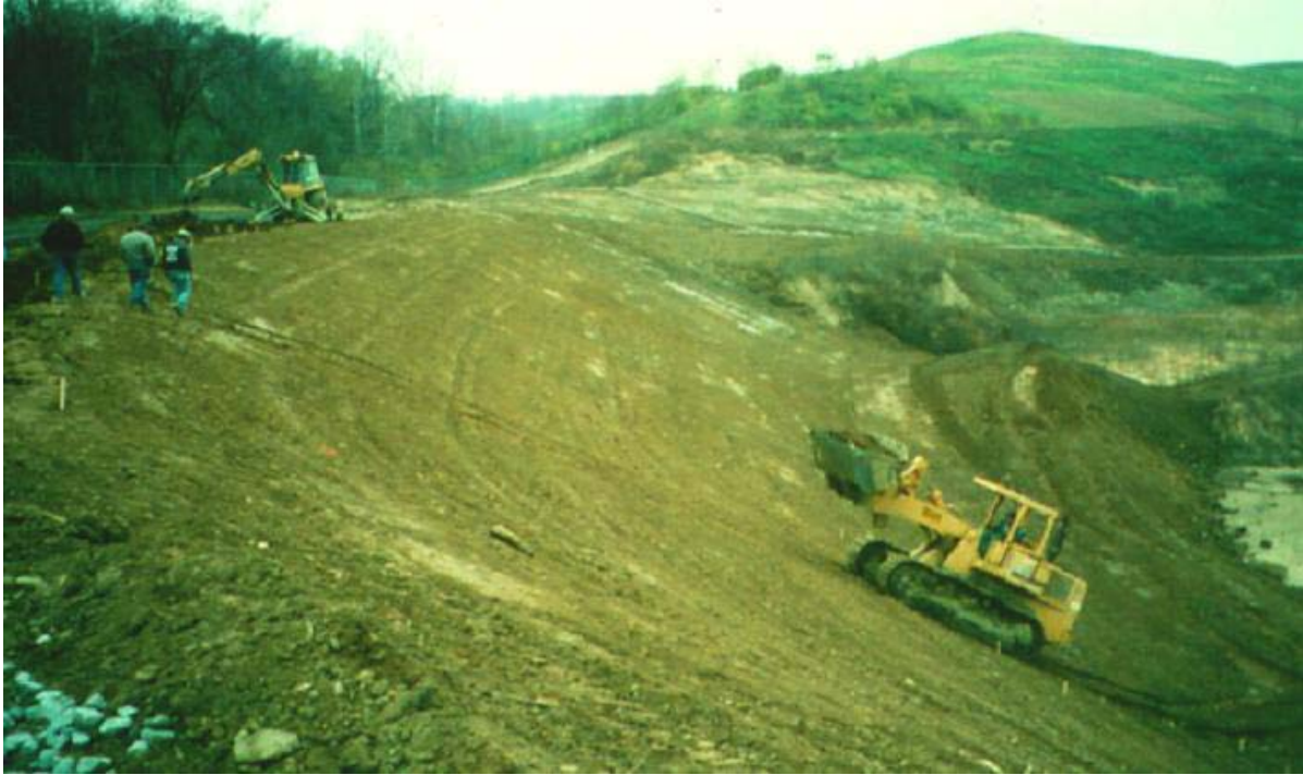
Figure 3-11. Prepared surface on which 2H:1V test plots were constructed.
