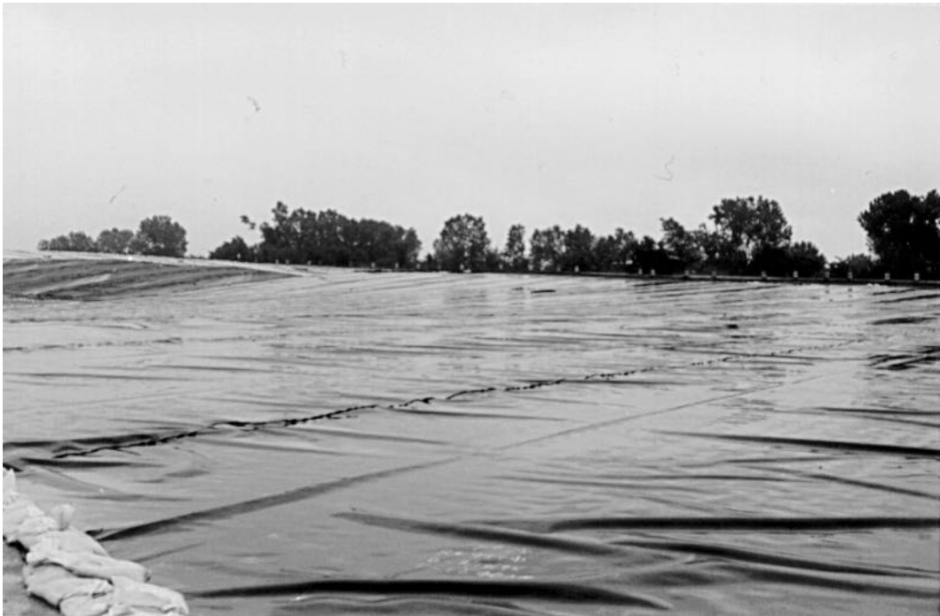
Figure A-1. Relatively small waves, or wrinkles, in a field deployed GM.
