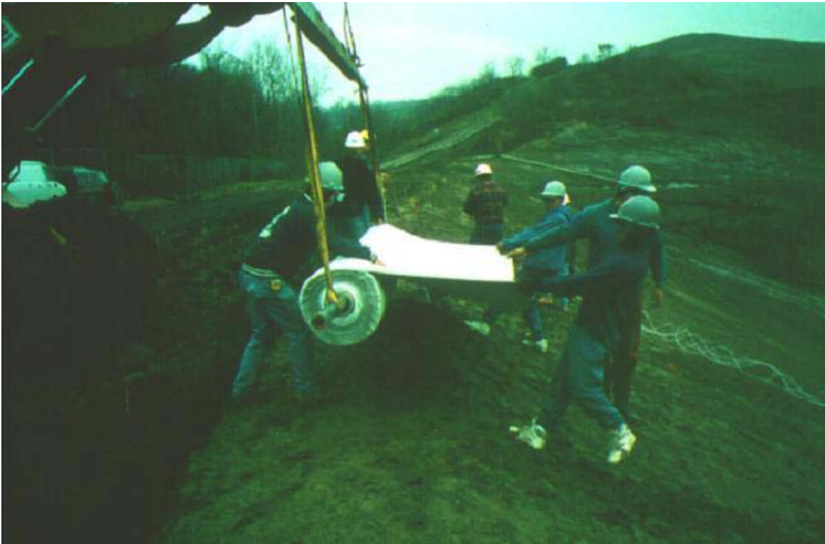
Figure 3-12. Typical installation of geosynthetics.
