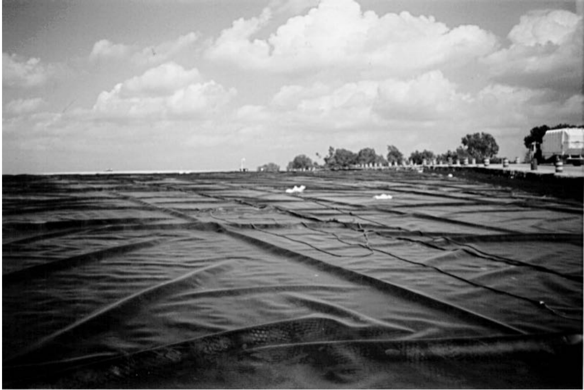
Figure A-2. Relatively large waves, or wrinkles, in a field deployed GM.
