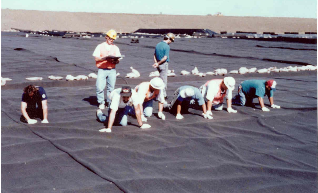
Figure F-A.4.1. Manually searching for needle fragments in an installed GT.
