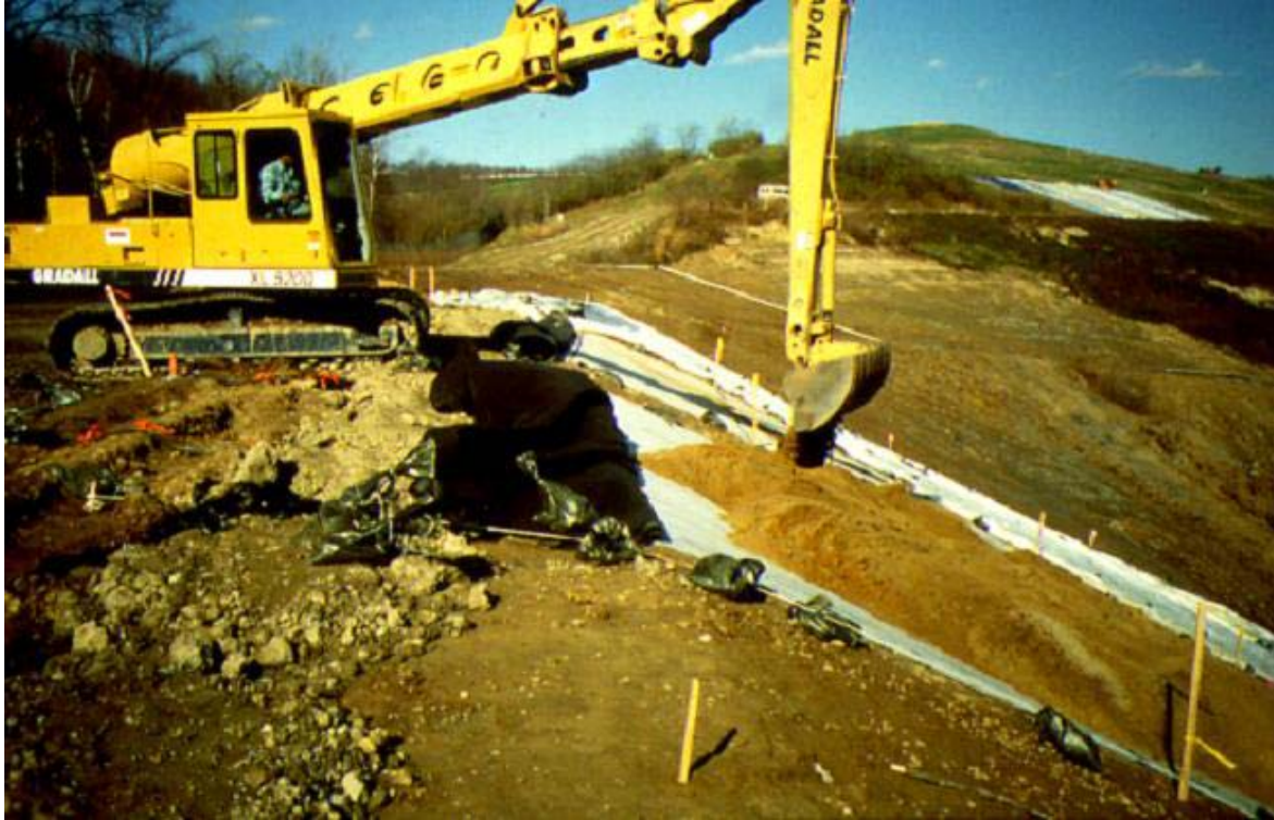
Figure 3-13. Placement of cover soil near top of slope.
