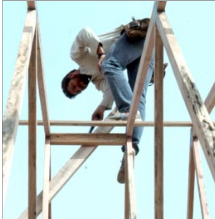
New safety guidelines under consideration by OSHA would affect procedures like truss erection, where current rules are said to be impractical.
