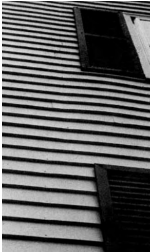
Figure 1. This hardboard has absorbed excessive moisture and expanded, causing buckling and bowing. Note how tight and swollen the butted joints are.
