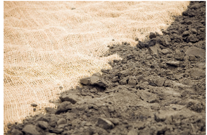
Geotextile matting protects bare soil from erosion caused by wind and stormwater.
