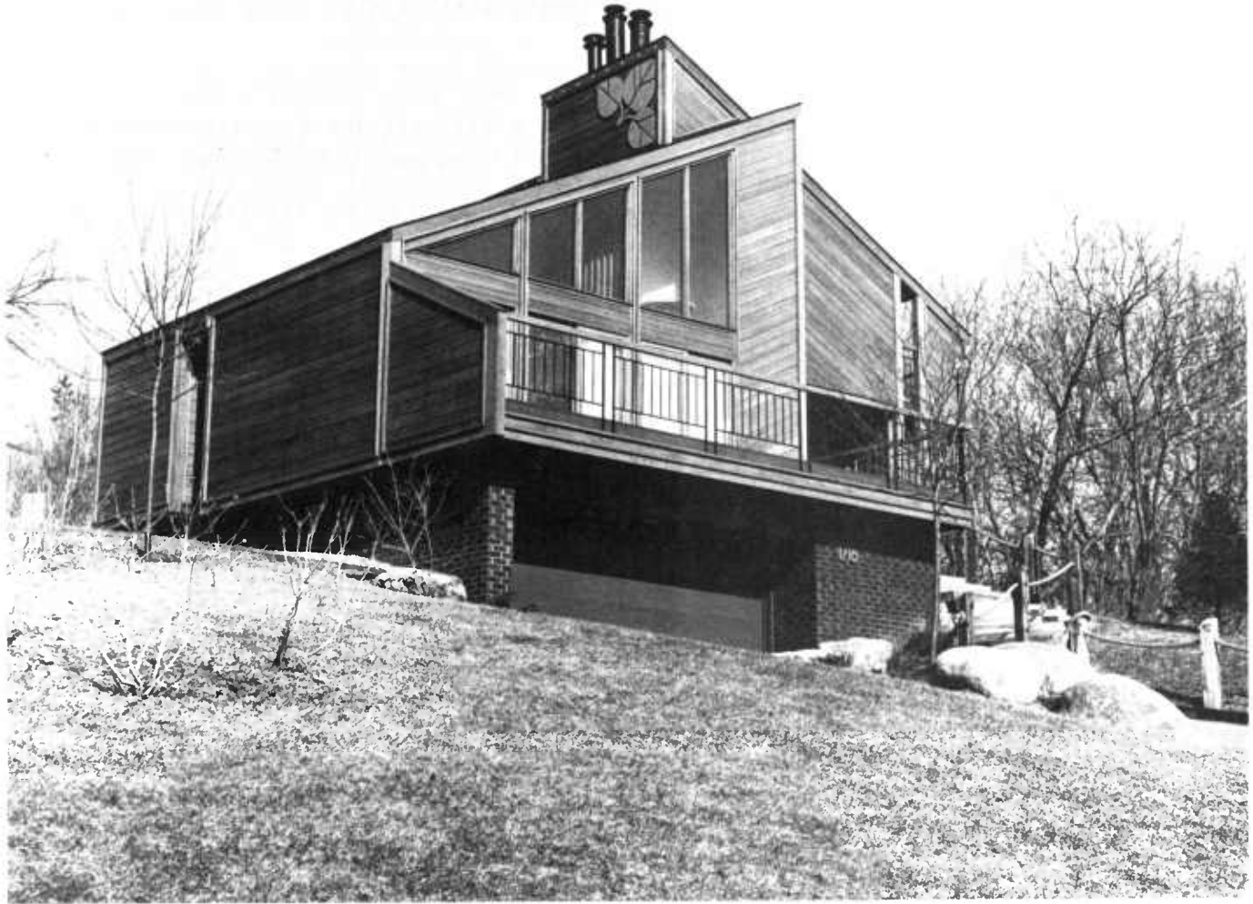
Figure 24 —Modern house finished with a semitransparent penetrating oil-based stain.
