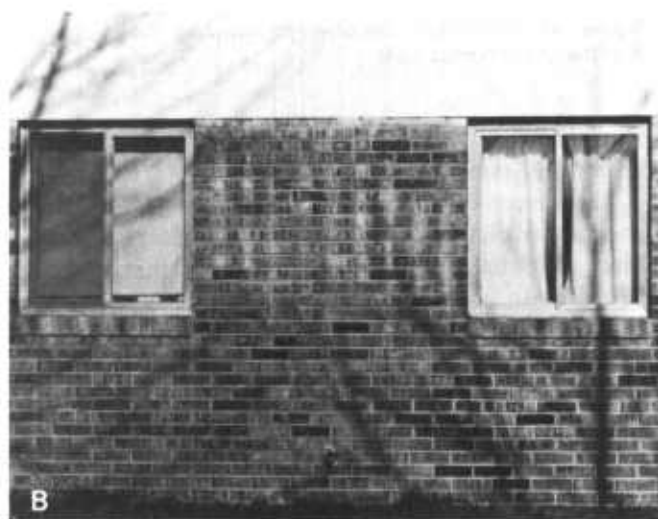
Figure 37 —Some paints or stains chalk badly and can discolor a lower surface as they wash down over it (A and B).
