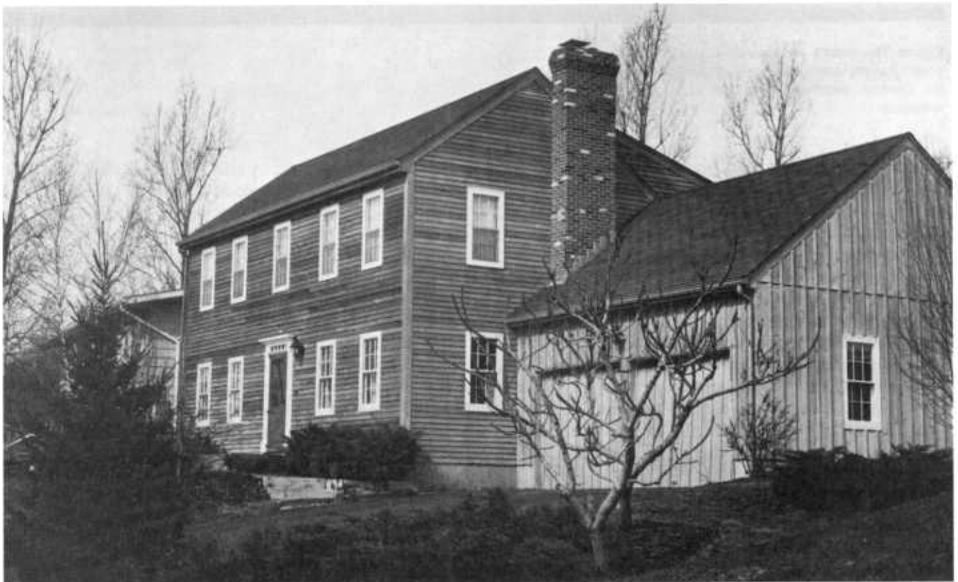
Figure 17 —House with western redcedar siding that has been allowed to weather naturally.
