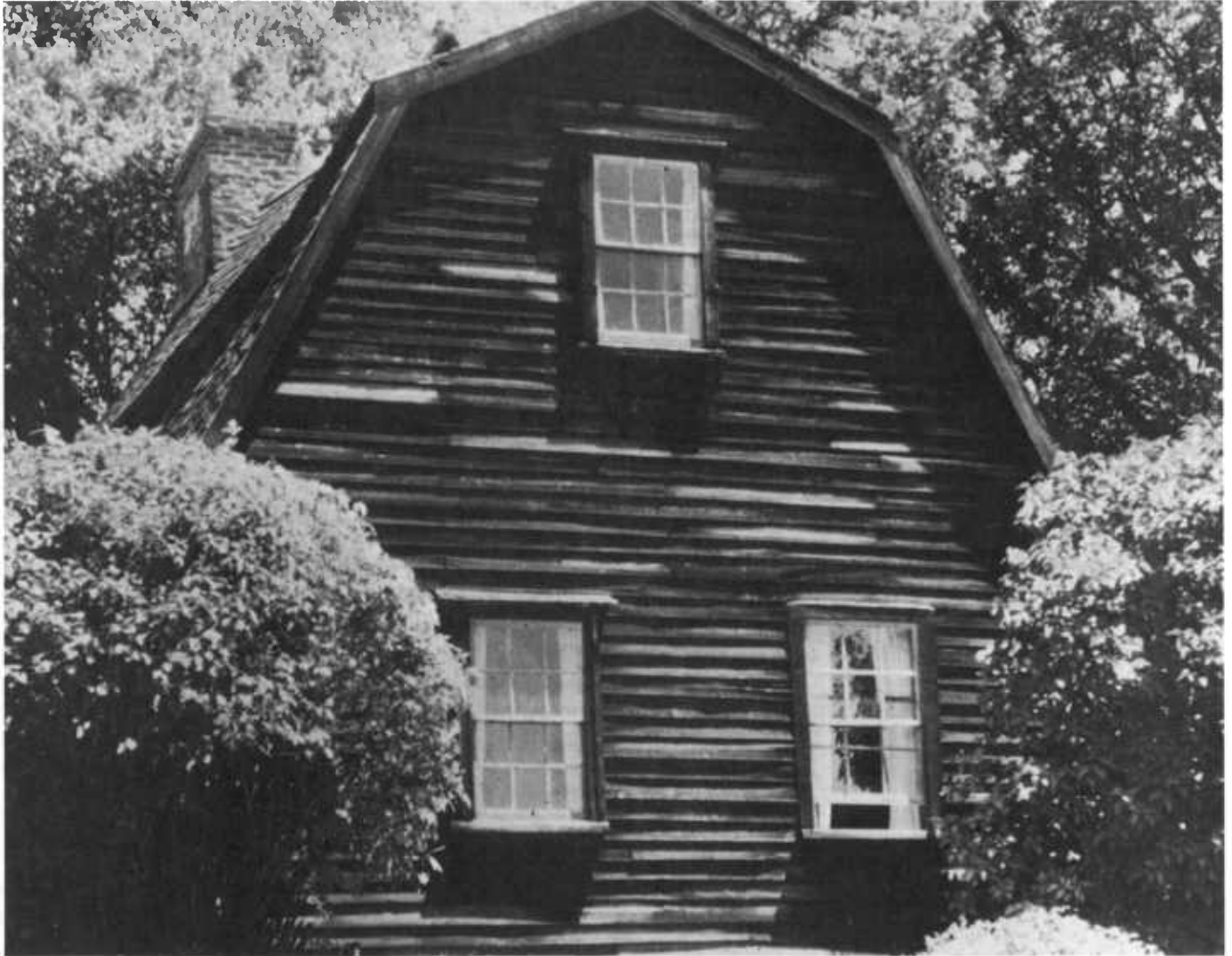
Figure 14 —Old Fairbanks house at Dedham, Massachusetts, built in 1637. Most of the white pine clapboard siding was replaced in 1903 and has stood 80 years without paint.
