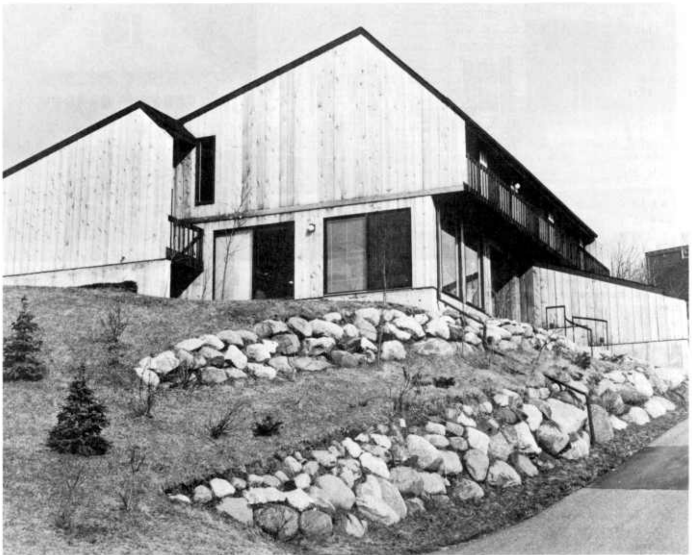
Figure 21 —Modern house with a natural water-repellent preservative finish.
