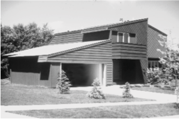
Figure 2—Structure finished with a semitransparent stain.
