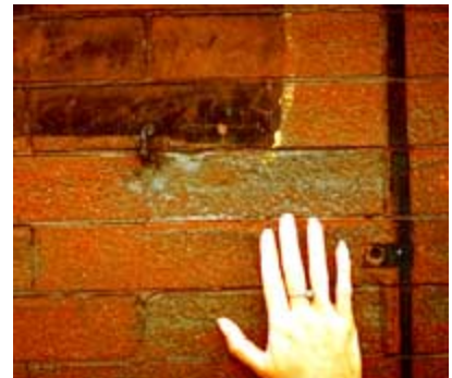
Undamaged historic brick (above). Sandblasted brick (below). Photo: Courtesy, Illinois Historic Preservation Agency.
