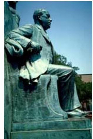
Bronze statuary may be cleaned gently using crushed walnut shells. Photo: NPS files.
