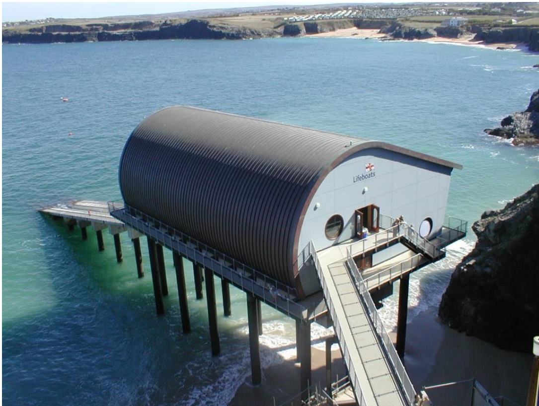
Figure 3.10. Padstow lifeboat station. Photograph by Benjamin Evans.
