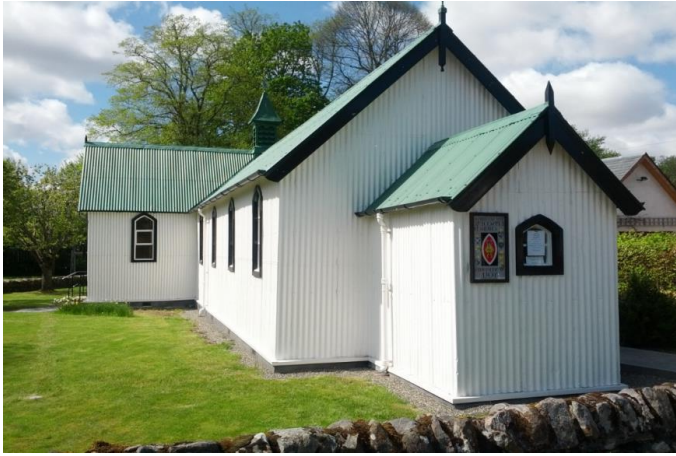
Figure 4.23. St Fillan's Chapel, Killin, after repair in 2014.
