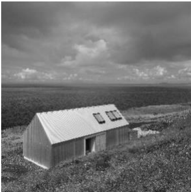
Figure 3.15. 'Tin House': functional corrugated iron is used by Nick Thomson as a main component of a house on the Isle of Skye. However, the apparent concentration on functionality is also a style statement because the building consciously echoes the Highland tradition of prefabricated corrugated iron. Photograph by Nick Thompson.
