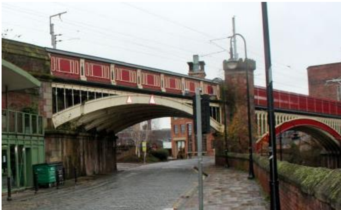
Figure 4.7. Castlefields Viaduct, Manchester: an example of ET Bellhouse's familiarity with cast iron engineering. Image from 'Castlefield Viaducts (Manchester),' Grace's Guide to British Industrial History , accessed 13 August 2019, https://www.gracesguide.co.uk/Castlefield_Viaducts_(Manchester) .
