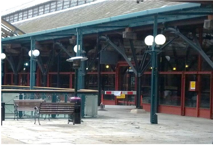
Figure A.6. The Tobacco warehouse at the London dock showing the early structural ironwork. The branching supports towards the back of the building is the iron installed by architect Daniel Alexander in 1811–14. Photograph by the author (2012).
