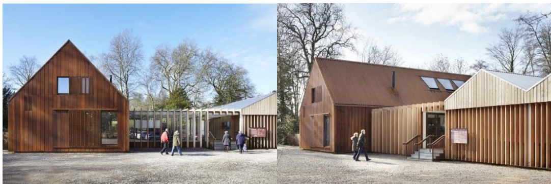
Figure 3.13. A successful use of Corten and corrugated iron at Mottisfont Abbey, designed by Burd Haward architects.
