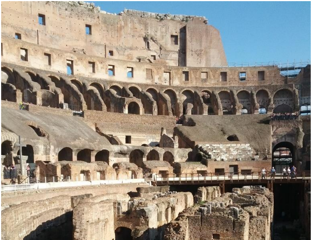
Figure 3.4. The Colosseum, Rome. The architecture visible in this image is composed of a random mixture of stone, brick and concrete, highlighting the indifference of Roman builders to stone: they simply used the cheapest and most adaptable material in any given circumstance. In reality the classical buildings were often not made from stone, but a mixture of brick, concrete and stone. Even the much-revered Palladio in the fifteenth century did not build from solid stone. His valorisation of classical architecture in the Italian town of Vicenza is largely built from brick and covered by imitation stone. Photograph by the author.
