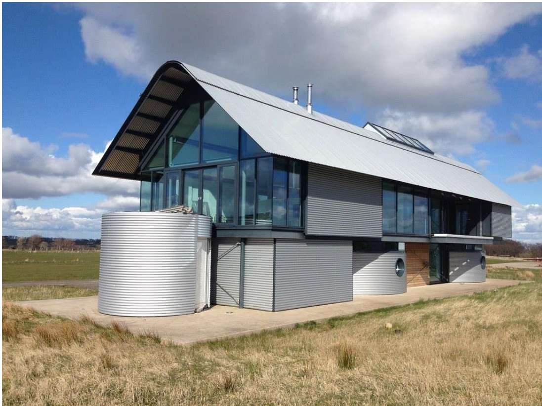
Figure 3.9. Strathaven Airfield House designed by Richard Murphy. Image reproduced with permission.
