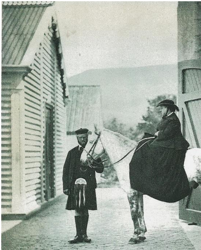
Figure 4.8. Queen Victoria on her horse with John Brown. The ballroom is to the left. The apparent age of the queen and the presence of John Brown implies that this photograph was taken in the 1890s. By this time the new castle including the ballroom had been completed and it is likely that Bellhouse's ballroom had been moved to its current setting. Image from Ivor Brown, Balmoral: The History of a Home (London: Collins, 1955), 113.
