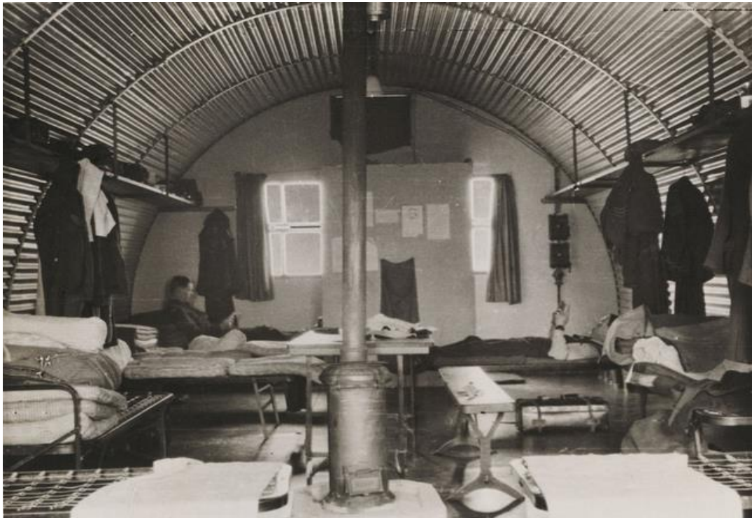
Figure 4.62. The lack of insulation in Nissen's design makes condensation on the inner faces of the hut unavoidable, thus damaging the fabric of the hut itself and making any productive use problematic. The picture illustrates the incompatibility between the conditions that were acceptable to the military during the Second World War, and modern demands for a satisfactory accommodation. Image from Australian War Memorial, accessed 23 August 2020, https://www.awm.gov.au/collection/C1276130 .
