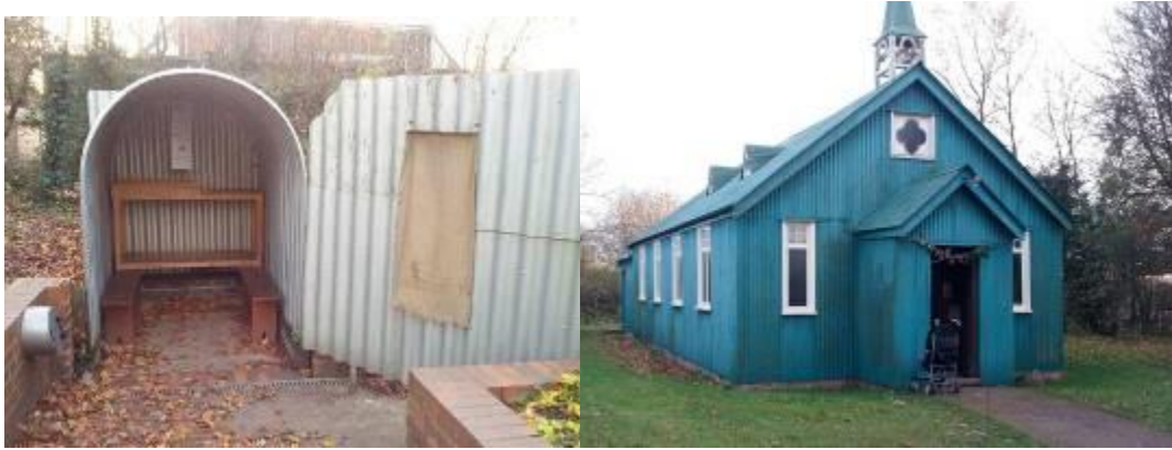
Figure 4.77. Avoncroft Museum of Historic Buildings. Left , the Anderson shelter. Right , the corrugated iron chapel. Photographs by the author.
