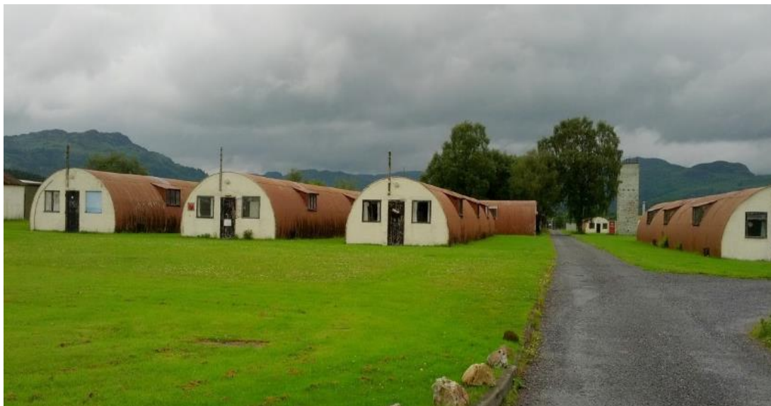
Figure 4.45. Cultybraggan POW Camp. This image gives some indication of the scale of the Camp. Photograph by the author.
