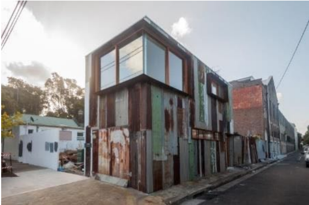
Figure 3.12. 'Tinshed,' Australia, designed by Raffaello Rosselli. In an unusual decision, Rosselli has used the material in its broken and battered form. Apparently, when the builders finished the initial build, he felt it was not battered enough and adjusted the sheet of corrugated iron to make it look wobblier. Perhaps it should be no surprise that this exciting use of corrugated iron is being created in Australia. Image reproduced with permission.
