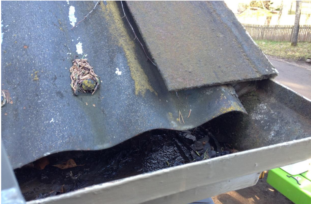
Figure 4.10. Balmoral ballroom guttering. Photograph by the Factor of Balmoral, 2014.
