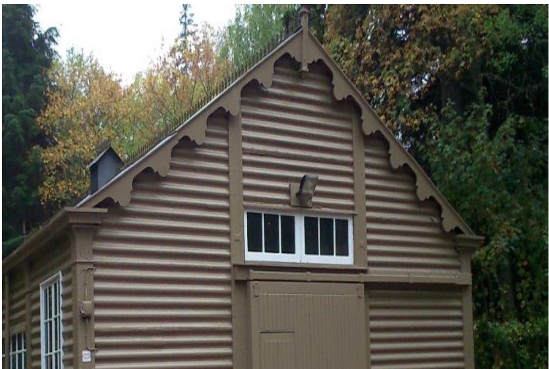
Figure 4.16. The most significant external details are the cast iron framing and the original corrugated wrought iron panels, but additional details include the decorative barge boards, and roof detailing with an elaborate ventilator and cast iron brattishing along the crest. It is unclear if these details have been replaced, but they are in excellent condition.
