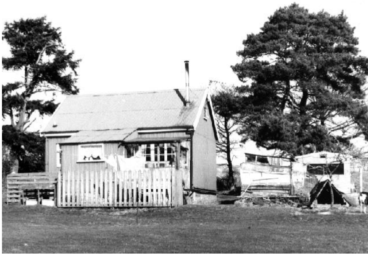
Figure 4.21. The Shooting Lodge, Morden, Dorset. This cottage, much loved by its occupiers, started life as a shooting lodge in a different location. The owners have demonstrated that ingenuity is one of the most important elements of adaptability by reusing the old corrugated iron from removed during roof repairs by making it into a new goat shed.
