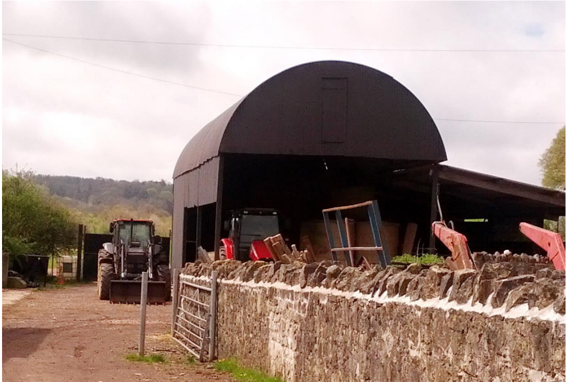
Figure 4.66. The barn at Llwyn yr eos Farm, St Fagans, Cardiff. Agricultural buildings such as these were mass produced in the nineteenth and twentieth centuries and survive in very large numbers. Because they are so numerous and utilitarian, they have had a major role in influencing perceptions of the significance and value of all corrugated iron buildings. Photograph by the author.
