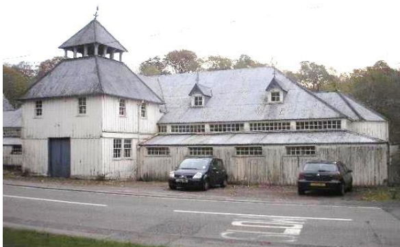
Figure 4.2. Drill Hall, Golspie, Sutherland. One of the fascinating deployments of corrugated iron that was impractical as a case study. The image was taken in October 2009 and the condition has deteriorated significantly since then. The Drill Hall is a striking example of how difficult it can be to find truly beneficial re-use for buildings that were created to fulfil highly specific uses.
