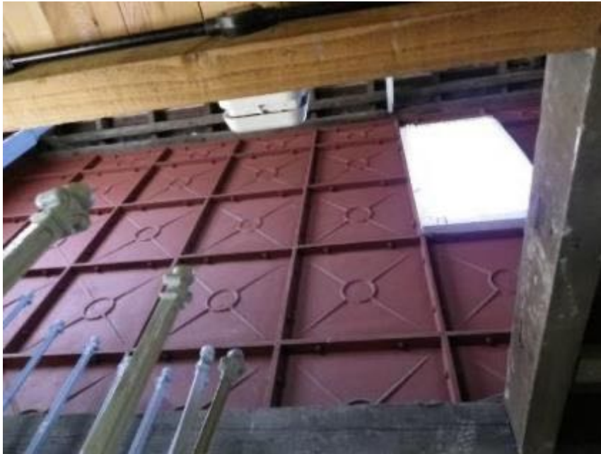
Figure 4.3. The wall of a house at the Black Country Museum – made from cast iron tiles. Metal buildings have never been as economical to building compared with other materials.
