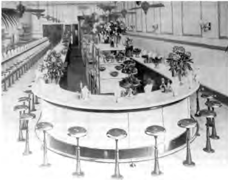
Structural glass was popular in restaurants due to its sanitary, non-absorbent and non-staining qualities. This restaurant had Carrara and Black Glass walls, wainscoting, counters, aprons and shelving. Source: Glass, Paints, Varnishes and Brushes: Their History, Manufacture, and Use, 1923.
