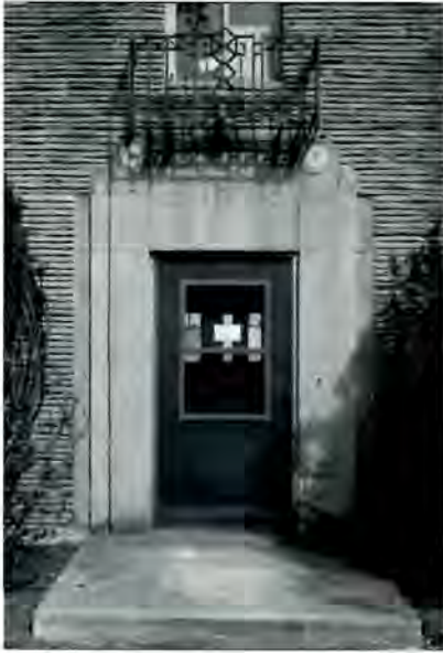
The door surround on the Wieboldt-Rostone House (Walter Scholer, 1933) is the only area of the exterior where the original building material, Rostone, a precast form of simulated masonry, is intact.
