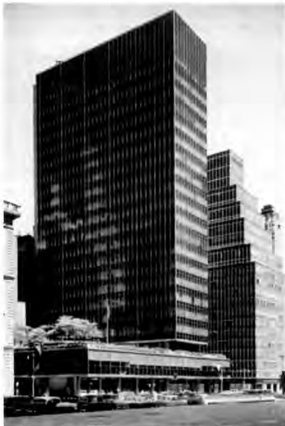
Fig. 2. Lever House, New York, New York (Skidmore, Owings and Merrill, 1952). The clean curtain wall appearance "belies its complex internal construction which was cobbled together from off the shelf parts," as described in Architectural Record , June 1989.
