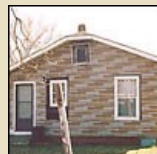
The popular 1950s look of cut sandstone could be achieved through the inexpensive application of Ranch Stone asphalt siding.
