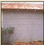
Asphalt rolls that imitated irregular courses of cut stone could be purchased by the early 1940s.
