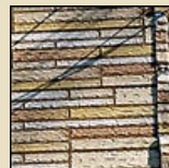
Mid-1960s Random Stone was similar to Ranch Stone but it featured a wire-cut brick shape among the "courses" of stone shapes.
