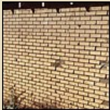
Asphalt strip shingles in imitation of brick hit the market in the early 1930s.
