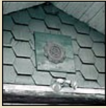
Asphalt hexagonal shingles were used as alternative wall coverings in gable ends and dormers.
