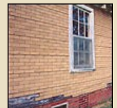
Rolled asphalt brick siding was made possible through the introduction of heated rollers that pressed patterns into the surface.
