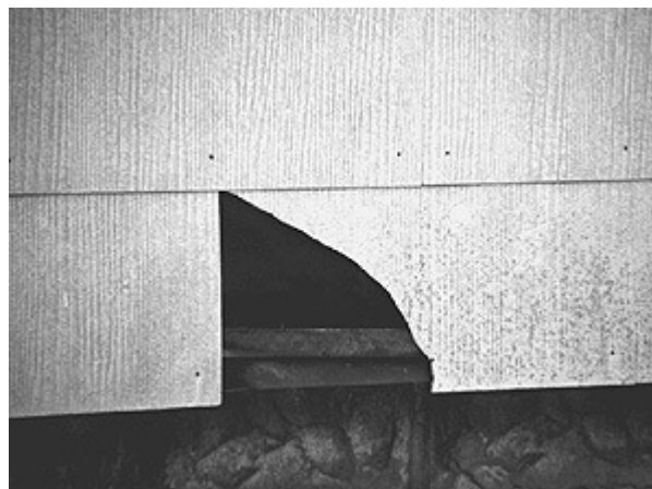
Figure 6. Asbestos-cement products most commonly deteriorate by cracking and chipping. These kinds of deterioration are not typically feasible to repair, and therefore it is recommended that a non-asbestos fiber cement piece be used as a replacement (photo by author).
