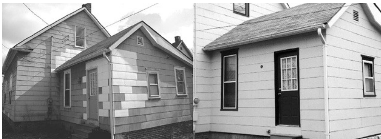
Figure 7. Replacement non-asbestos fiber-cement shingles in place, before being painted and after (photo by author).
