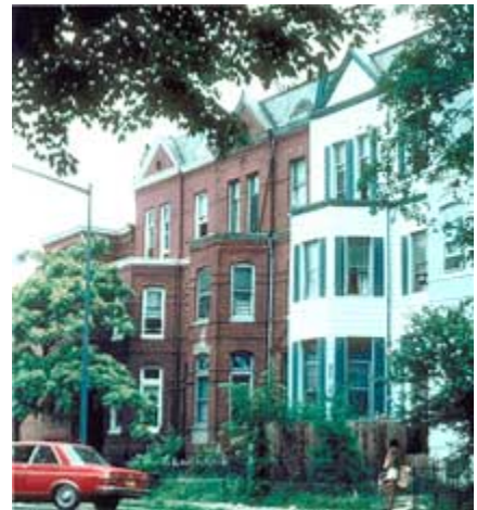
The inappropriate siding applied to the house on the right has altered the character of the urban setting. Photo: NPS files.
