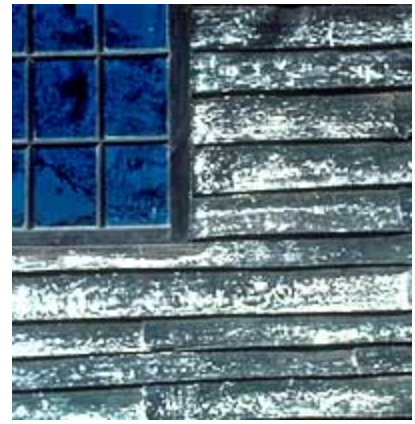
Historic wood siding exhibits rich and varied surface textures. They range from hand-split clapboards of short lengths with feather-edged ends (shown here), to pit or mill sawn boards which can be beveled, rabbeted, or beaded. Photo: NPS files.
