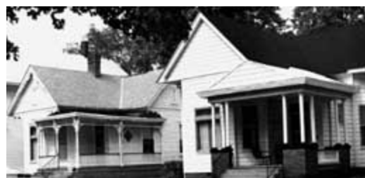
When aluminum was installed on the house on the right, the barge boards, scrollwork, columns, and railings were removed. The distinctive shingled gable and attic vent were covered, further compromising the building's architectural integrity. Photo: NPS files.
