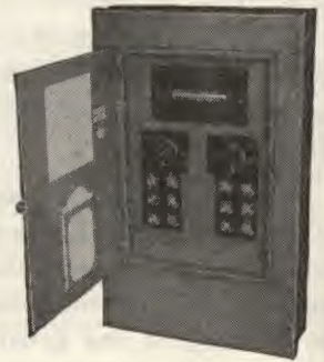
Fig. 7-3. A larger switch. Besides main fuses it has plug fuses for twelve 115-volt circuits, and cartridge fuses for two 230-volt circuits.
