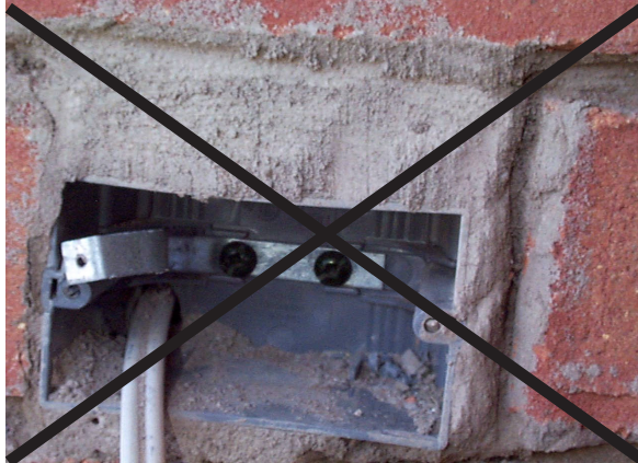
Photo B2 – A conductor that is not protected from sharp edges; non-Code compliant installation
