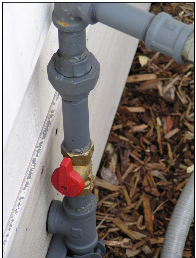
Figure 2-5 Manual Fuel Shutoff Valve (outdoor installation shown)
