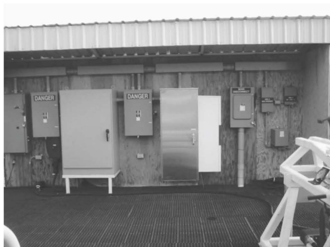
Fig. 3. Electrical supply for the motor testing
