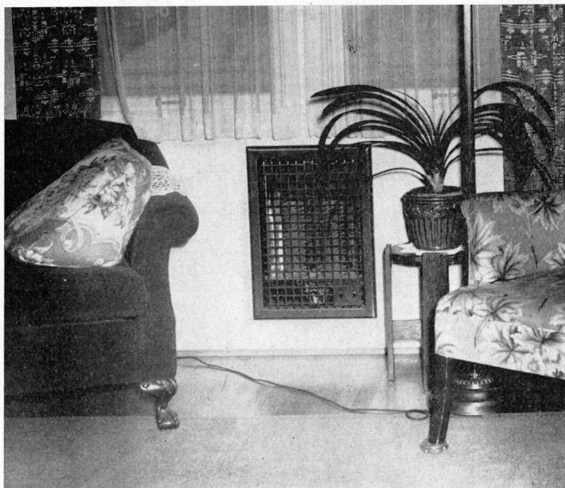
Figure 2. AN ELECTRIC RADIANT-CONVECTION UNIT HEATER INSTALLED.
