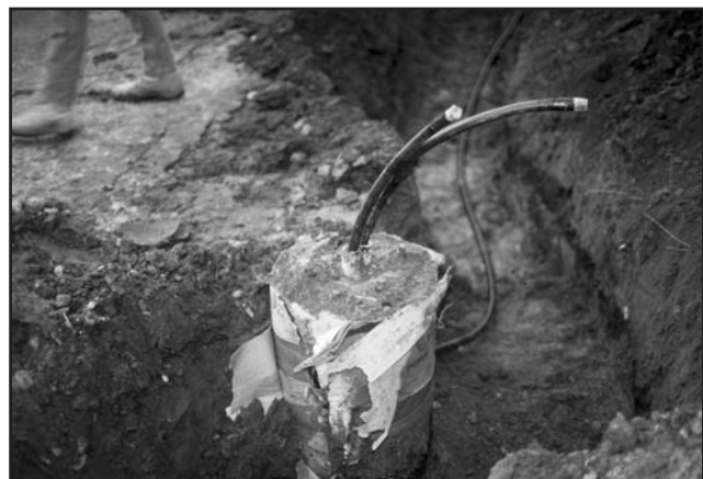
Figure 5.3.2—PVC Jacketed Cable (courtesy AFC Cable Systems)
