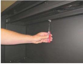
The fireback clip has a keyhole slot. It can be removed by loosening the screw and sliding the clip out.
