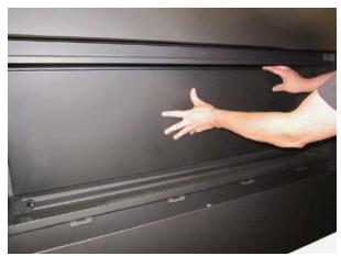
4 Replace the rear fireback clips to secure the rear fireback in place.
