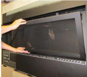
3. Use the glass tool to unlatch the glass frame. Remove the glass frame. The glass frame is held in place with four tabs inserted into four slots at the bottom of the firebox opening.
