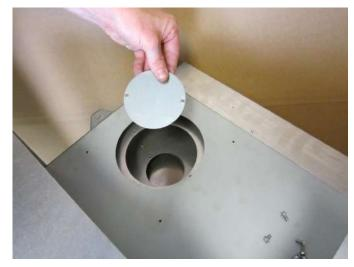
4 Loosen the single screw on the convection cover plate two turns.
