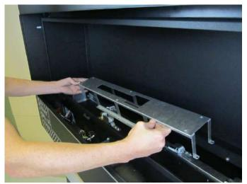
5. Remove and discard the NG (stock) manifold cover and orifice gasket (1/4" nutdriver). Install the LP manifold cover included in the owner's pack.
