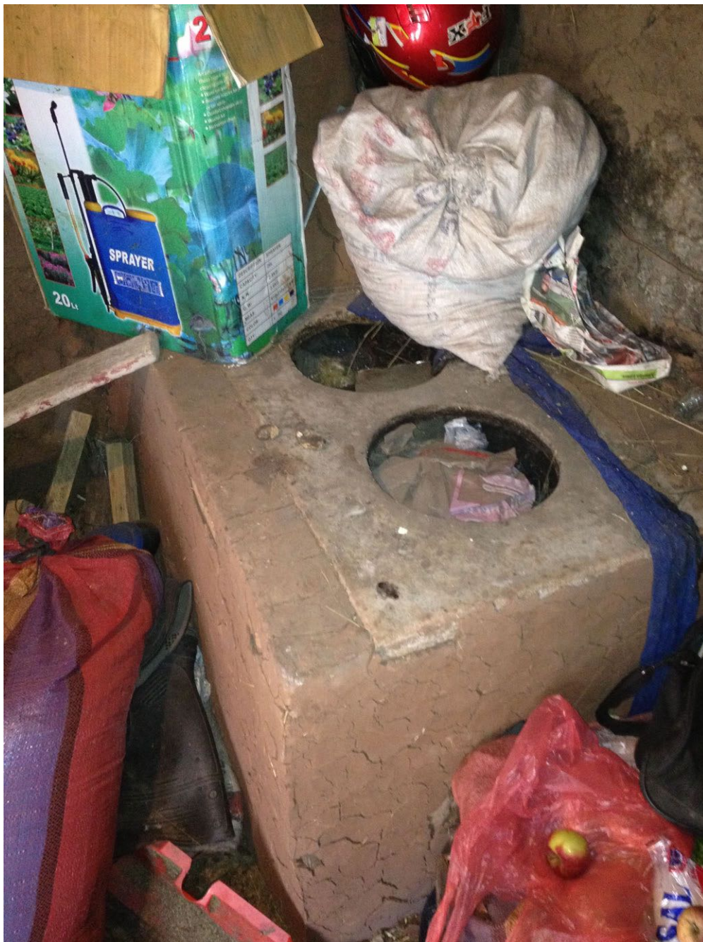
FIGURE 3. This InkaWasi stove, installed in 2011, had been converted to a makeshift food storage device less than a year after installation.
