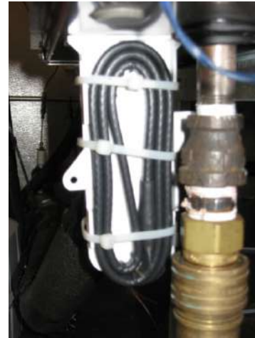
Figure 5. Heat tape on a condensate trap
