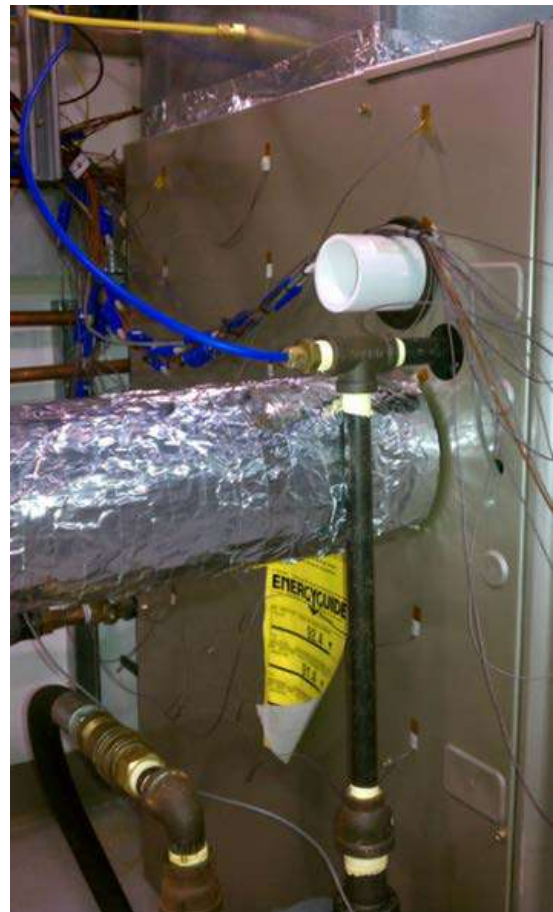
Figure 16. Furnace AFUE test showing jacket loss detail
