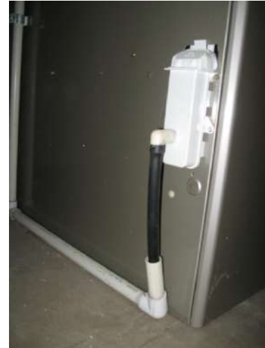
Figure 14. Verify that the condensate trap is working properly
