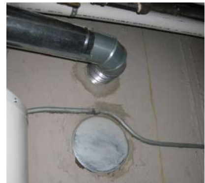
Figure 13. Seal unused vent openings
