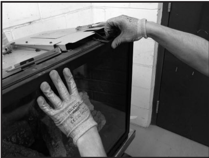
Figure 4.3 Release Glass Latches One at a Time
