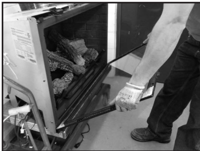
Figure 11.5 Tilt Glass Down and Lift Up to Disengage Bottom Latch
