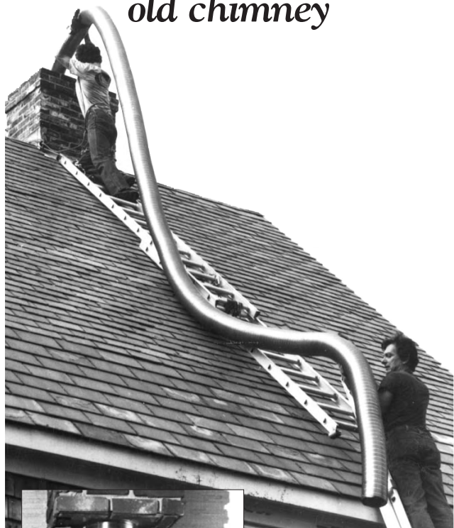
Flexible stainless-steel pipe is a good choice for lining an old masonry chimney. It comes in several alloys to match different fuel types, and it easily installs in any chimney configuration, even one with an offset (left).
