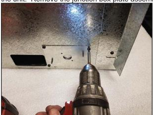
Remove the junction box coverplate. (2 screws)
