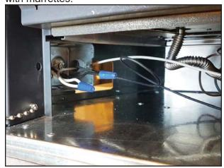
3. Coil the wires inside the junction box and refasten the cover plate.
