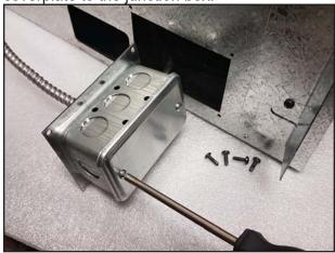
6. Refasten junction box assembly to the side of the appliance.
