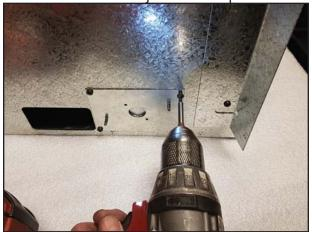
Remove the junction box coverplate. (2 screws)
