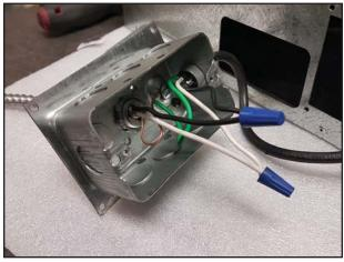
6. Coil wires and refasten junction box coverplate to the junction box.
