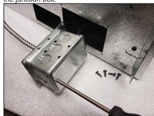
7. Refasten junction box assembly to the side of the appliance.
