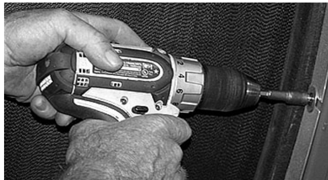
FIGURE 75 - LOOSEN SCREWS BEFORE ADJUSTING SEALS
