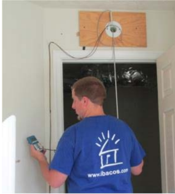
Figure 5. Measuring airflow rate using a hot wire anemometer
