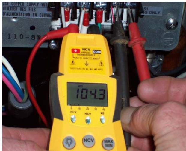
Outdoor unit at U1 & U2 communication line
