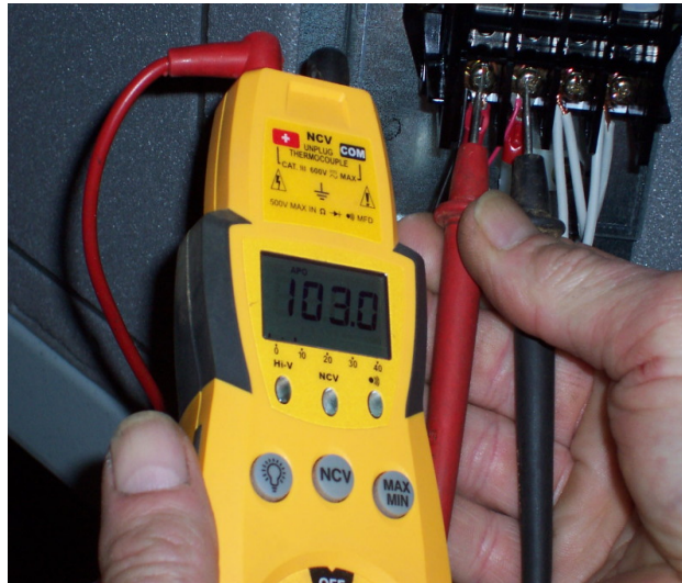
Outdoor unit at U1 & U2 communication line
