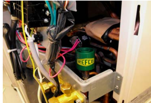
Place the tool over the EEV stem
