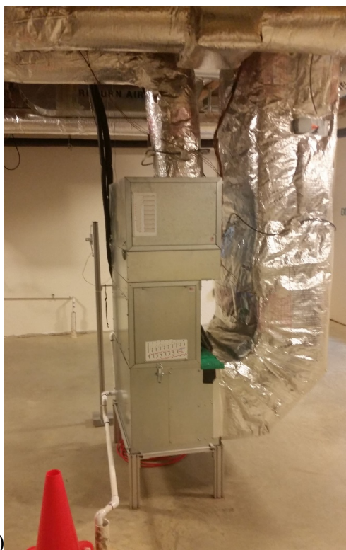
a) b) Figure 4: CDHP system indoor and outdoor units at the NZERTF, a) indoor air handler and b) outdoor unit
