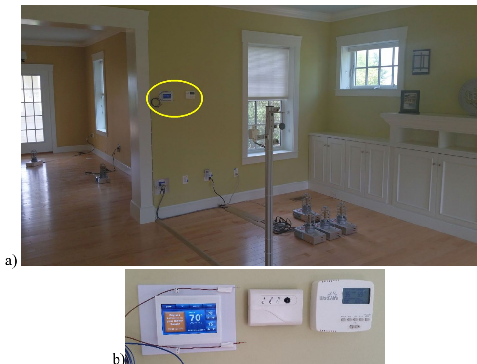
Figure 2: Thermostat locations, a) wide view and b) detailed view
