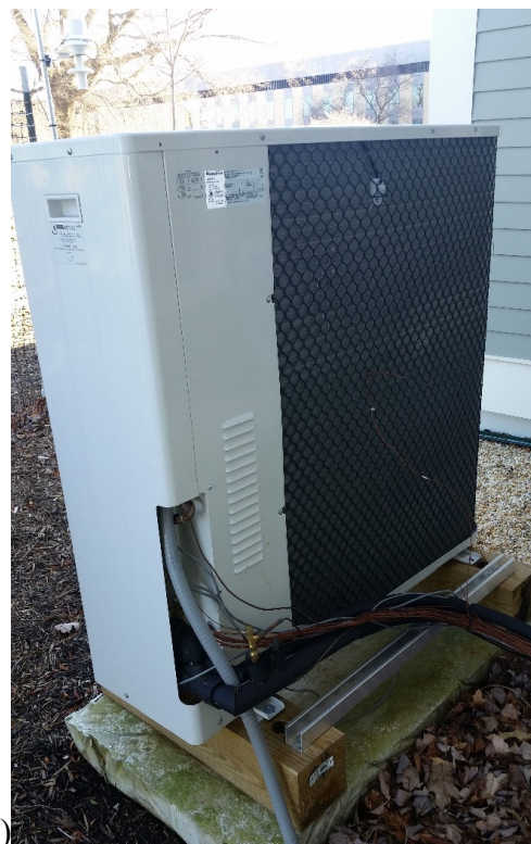
a) b) Figure 4: CDHP system indoor and outdoor units at the NZERTF, a) indoor air handler and b) outdoor unit
