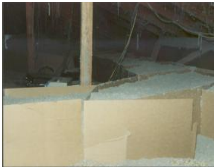
Blown -in insulation with cardboard forms
