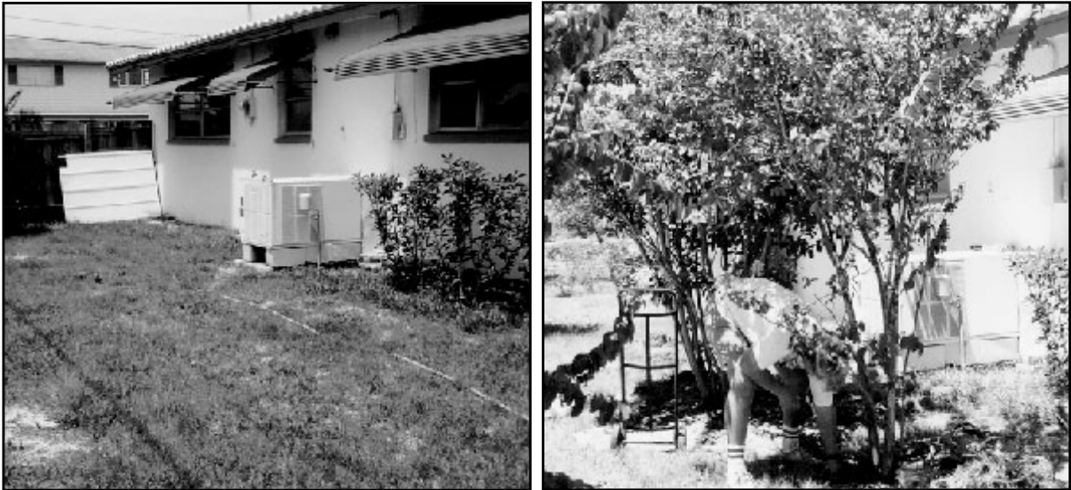
Figure 7. West-facing AC Condenser Shading at Site 3 before Landscaping (Left); Planting of Four Crape Myrtles for Shading (Right)
