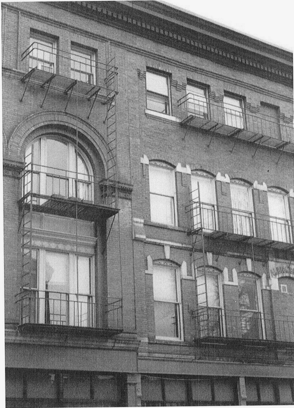
FIG. 2 Straight ladders between balconies, the type of fire escape commonly found on New York City tenements before 1900. (Photo by the author.)
