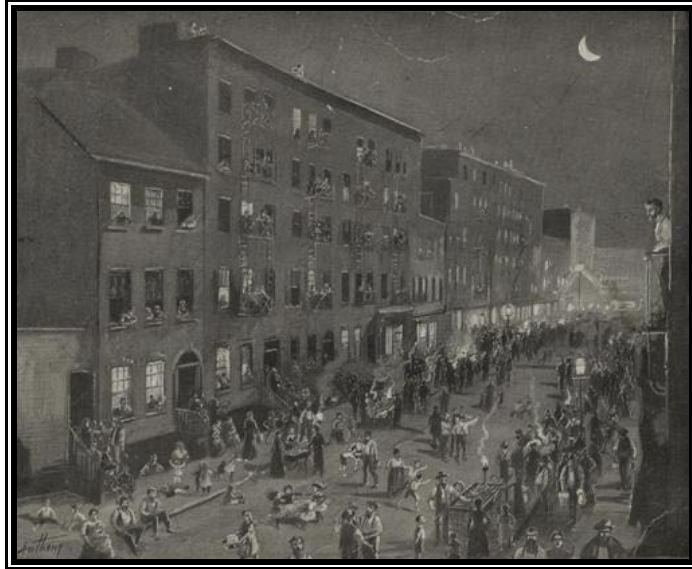
Figure 29: Tenement dwellers pour onto the streets and fire escapes for fresh air, Anthony, A Not Night on the East Side , 1899 (New York Public Library Digital Collection, Mid-Manhattan Picture Collection, Digital ID: 801547, http://www.nypl.org/digital/index.htm )
