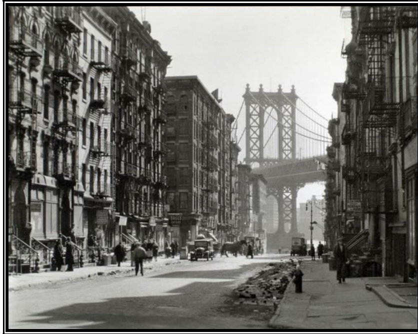
Figure 11: Tenement house façade lined with fire escapes. ( Pike and Henry Streets, Manhattan, 1936 , Berenice Abbott Changing New York Collection, Digital ID: 482697, New York Public Library Digital Archives, http://www.nypl.org/digital/index.htm )
