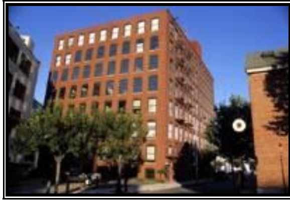
Figure 113: 150 Doran Building, Jewelry Manufacturing Historic District, Providence, RI. Fire escapes can be seen on the facade on the right (Providence Historic District Commission, “Design Guides for the Jewelry Historic District,” Providence, Rhode Island, http://www.providenceri.com/government/planning/historic/DownCity_regs.html )
