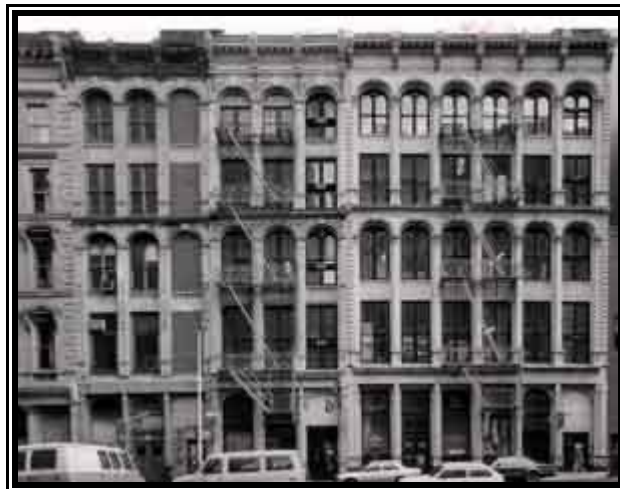
Figure 115: Historic TriBeCa block in New York City that maintains its fire escapes (Allen, Oliver E., “Architecture,” Tribeca Organization, http://www.tribeca.org/history/architecture.aspx )
