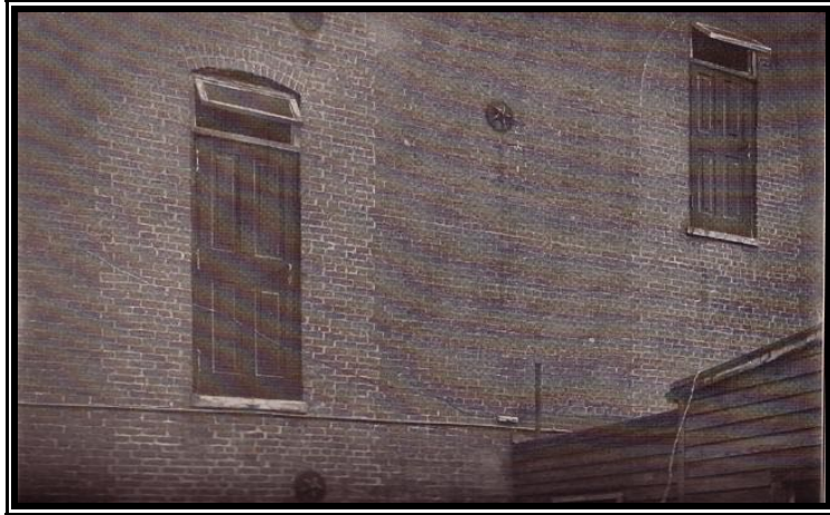
Figure 18: False exits on a Pennsylvania theatre. (“False Emergency Exits,” Quarterly of the National Fire Protection Association 9 (1916), 386.)
