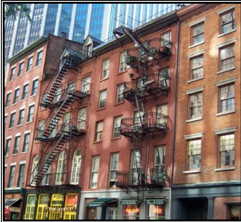
Figure 1: Fire escapes line historic buildings in Lower Manhattan in New York City. (author, 2004)
