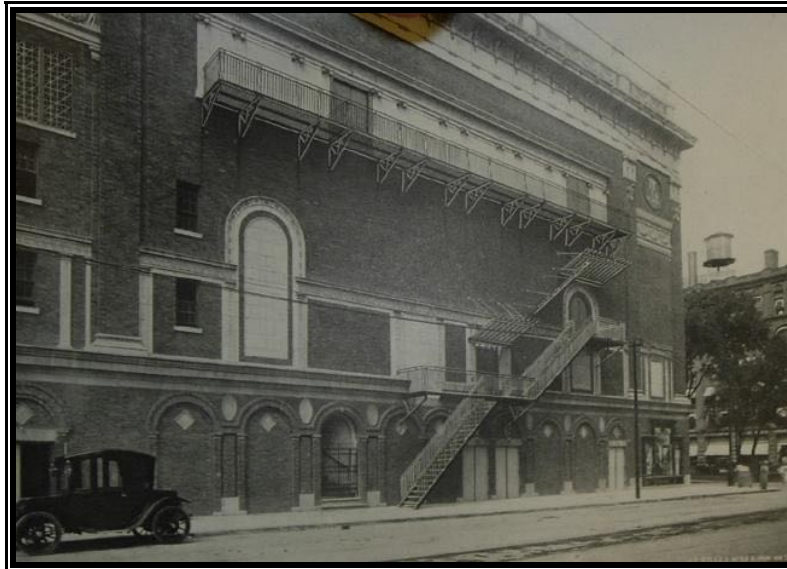
Figure 19: Demonstration of sufficient fire escapes on a Detroit, Michigan, theatre. (J.E. Bolles Wire and Iron Work. Sectional Catalogue . Detroit: The Firm, 1913: 89)
