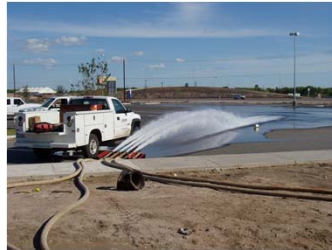
Photo courtesy of Protection Development Inc.
