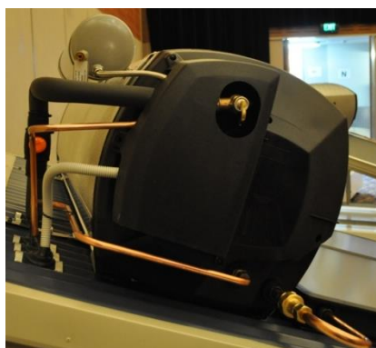
Installation of Pipe Shroud Cover with a HartStat Over Temperature Protection System
