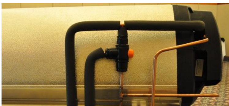
Installation of Pipe Shroud Cover without a HartStat Over Temperature Protection System
