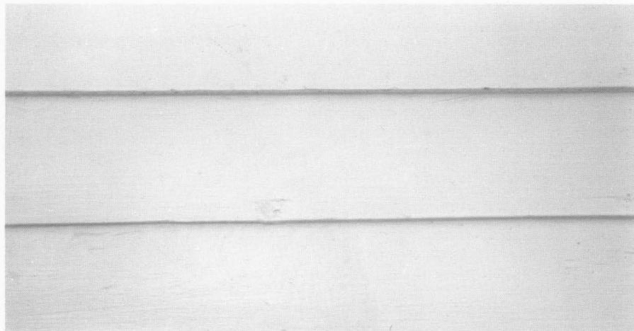
Figure 6. A typical section of the finish painted siding shows that little damage was done in removing the paint. Photo: Michael Lee
