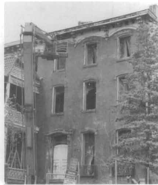
Figures 10a-10b. This test cleaning patch on brick and sandstone was allowed to weather over a full year, while other aspects of the rehabilitation were carried out. Finally the entire building was cleaned with a proprietary paint remover sprayed-on under low-pressure and then rinsed by workmen from a truck-mounted hydraulic platform lift.
