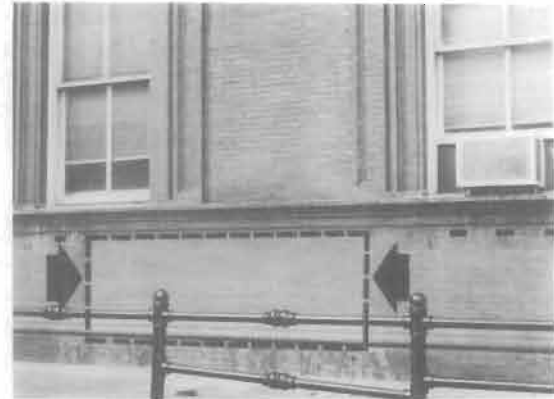
Figure 9. A test patch on brick to remove a century of dirt reveals only a slight difference in appearance between the cleaned and the uncleaned brick. The hard-baked outer skin of the brick provides a surface that is not only impervious to dirt penetration, but resists dirt accumulation. Photograph: Christina Henry
