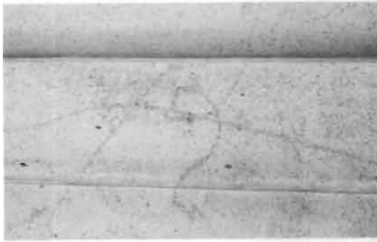
Figure 12. Water at too high a pressure from a pin-point nozzle has etched this white Vermont granite. Photograph: David A. Look, AIA
