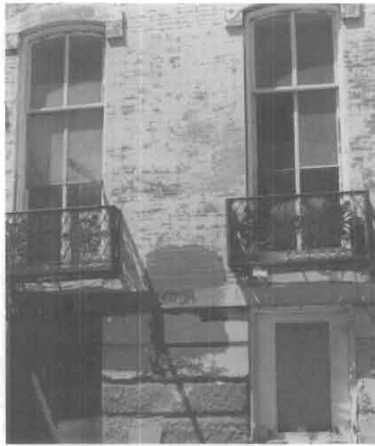
Figures 10a-10b. This test cleaning patch on brick and sandstone was allowed to weather over a full year, while other aspects of the rehabilitation were carried out. Finally the entire building was cleaned with a proprietary paint remover sprayed-on under low-pressure and then rinsed by workmen from a truck-mounted hydraulic platform lift.
