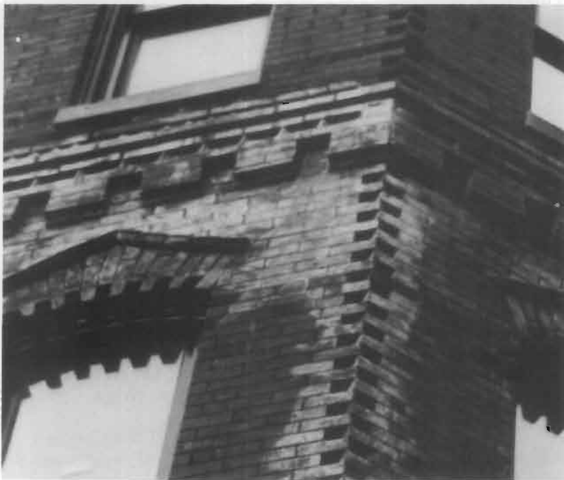
Figure 13. While hydrofluoric acid-based cleaners are often appropriate for cleaning unglazed brick, they may form hard-to-remove whitish silica deposits if left too long on the surface.
