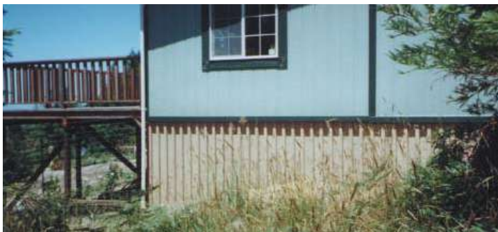
Figure 4.19 View site foundations (with decks) cost less.
