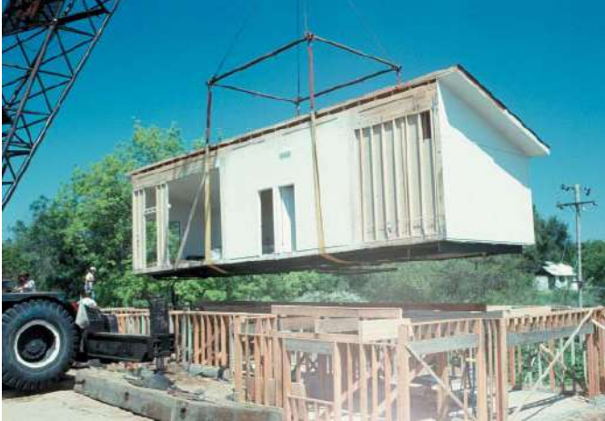
Figure 3.66 Above-ground basement with garage.
