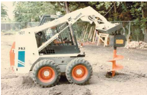
Figure 3.13 Digging chassis support footers with a power auger.
