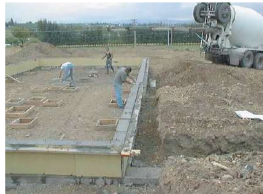
Figure 1.4 Some foundations are recessed to create a "site-built" look.
