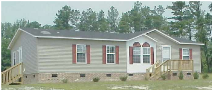
Figure 3.48 The access opening for this system is just behind the rear steps. Crawl space vents are evenly spaced in the foundation walls.
