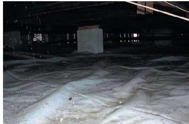
Figure 2.11 Polyethylene sheet for helping to keep moisture out of the crawl space.
