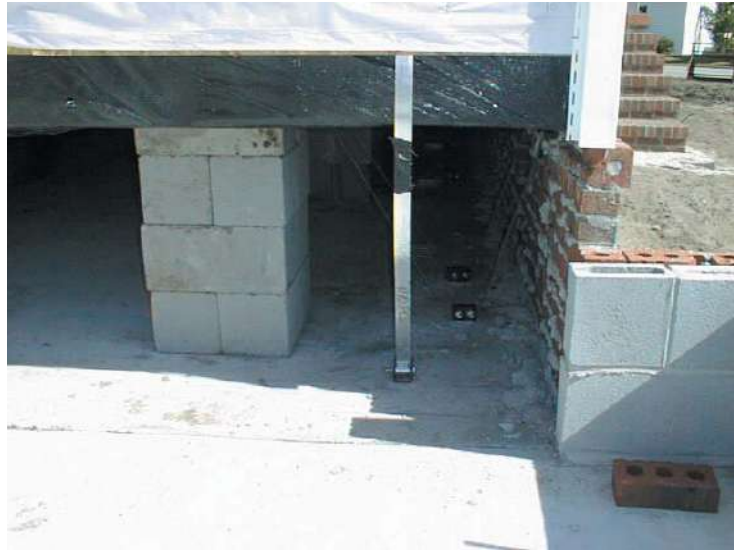
Figure 3.49 This view under a home shows block chassis supports, embedded anchors, and masonry exterior wall.
