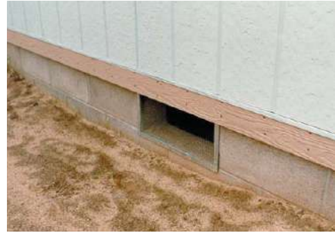
Figure 2.10 Foundation wall detail showing an air vent.
