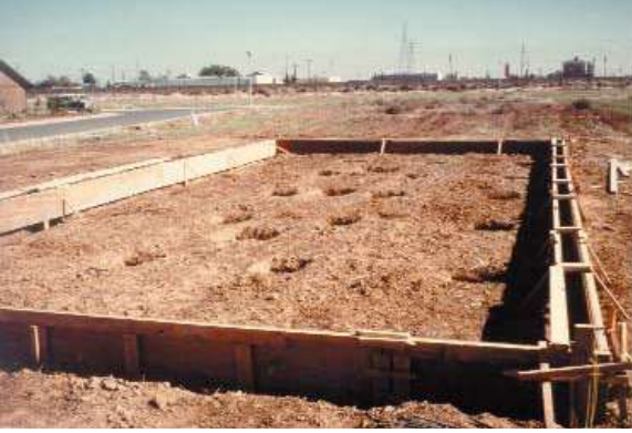
Figure 3.14 Forms ready for concrete pour.
