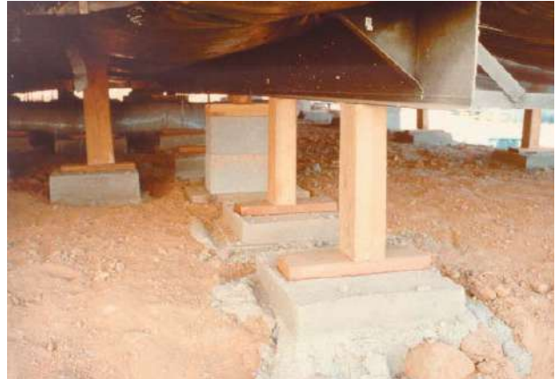
Figure 3.19 Economical support posts for chassis and ridge beam columns. Only used in conjunction with a structural perimeter wall.
