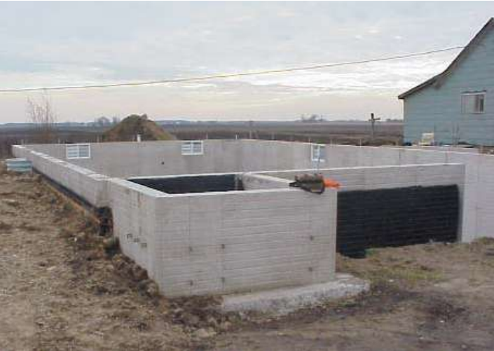
Figure 3.63 Basement showing backfill to create drainage slope.
