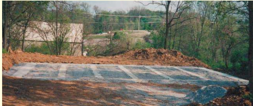
Figure 3.25 Open cells filled with crushed rock.
