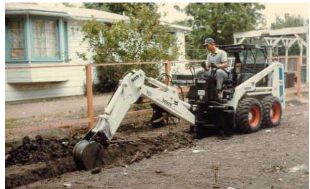
Figure 3.12 Excavating for perimeter footings with a backhoe.
