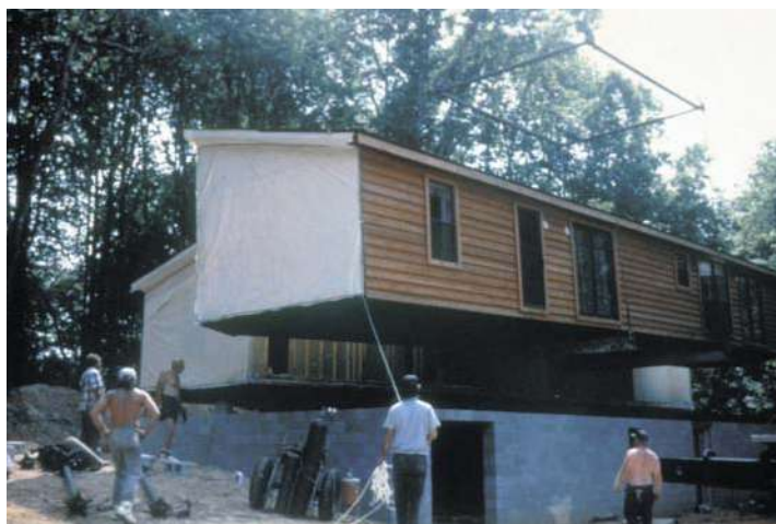
Figure 1.1 Crane set of a multi-section home on to a basement.
