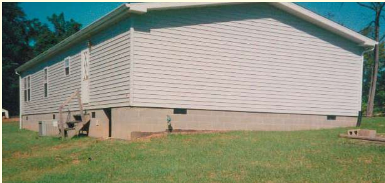
Figure 3.28 Nearly finished foundation system showing access door and crawl space ventilation openings.
