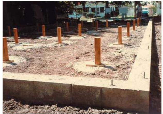
Figure 3.16 Carefully placed anchor bolts will not interfere with any portion of the manufactured home's floor joists.
