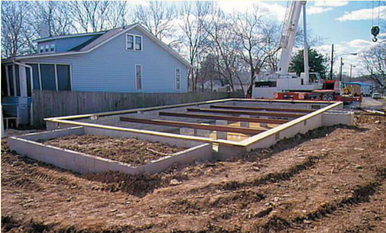
Figure 3.36 This foundation system, similar to the one used by Huddleston, is designed to carry the weight of the home at the perimeter and masonry walls.
