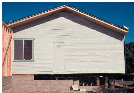
Figure 3.9 Stepped foundation.
