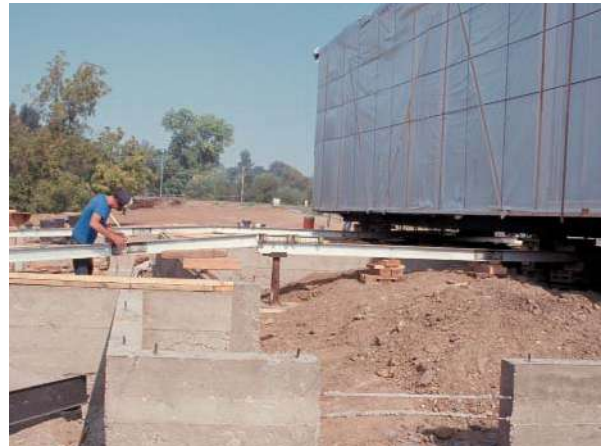
Figure 3.18 Installing a home with a roller system.
