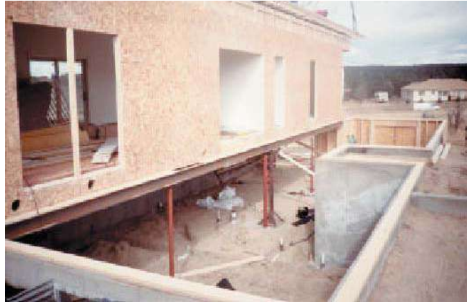
Figure 3.68 The structure of the basement includes supports for carrying the home at the perimeter and centerline.
