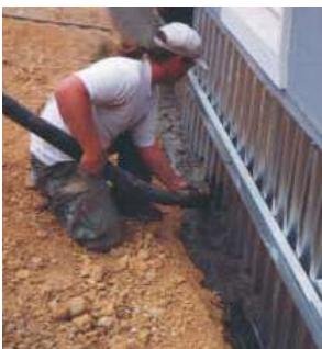
Figure 4.12 Concrete added to the trench.
