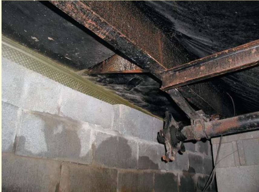
Figure 3.24 View of the Chateau foundation system from inside the crawl space.
