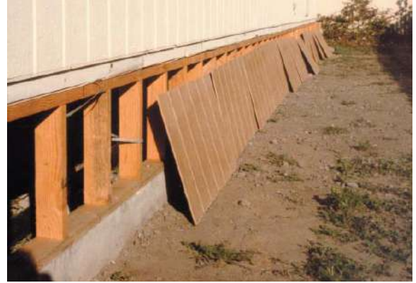
Figure 3.15 Ponywall construction method.
