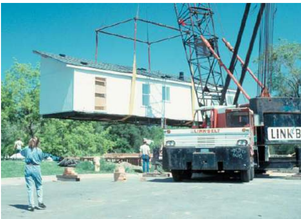
Figure 3.17 Installing a home with a crane.
