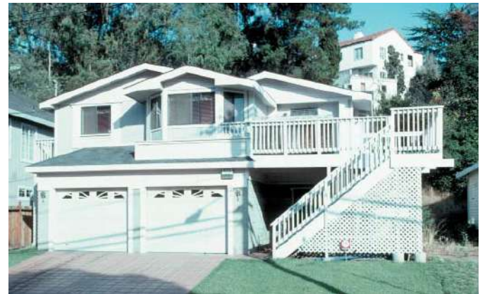
Figure 3.62 Garage/basement on upslope lot in Oakland, California.
