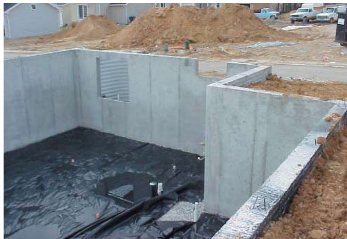
Figure 3.65 Basements are usually considered part of the living space and do not require vents for bringing in outside air.
