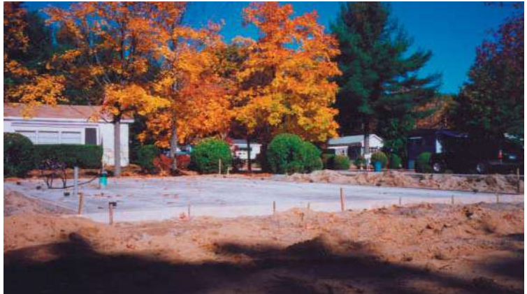
Figure 1.2 Slabs are an increasingly popular foundation system for manufactured homes, especially in the Northeast.
