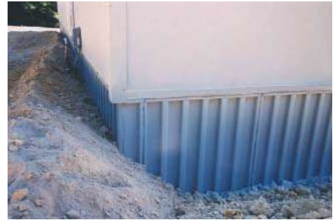
Figure 4.14 The coated panels can safely be backfilled.
